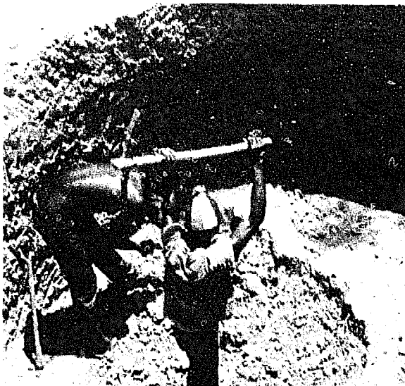
Photo 14: Excavation for a biogas plant (Source: OEKOTOP)
