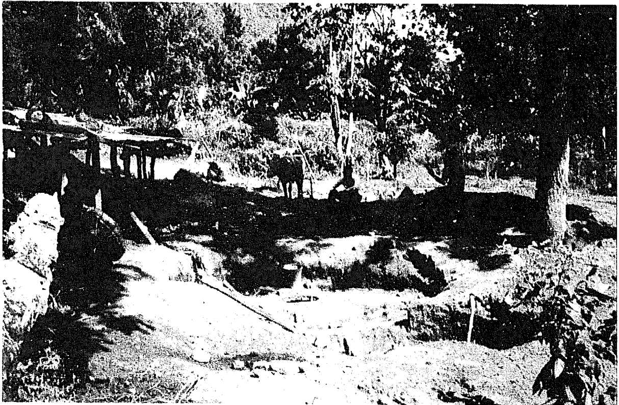
Photo 11: A nearly finished fixed-dome plant in combination with cattle shelter (Source: OEKOTOP, BEP Tanzania)
