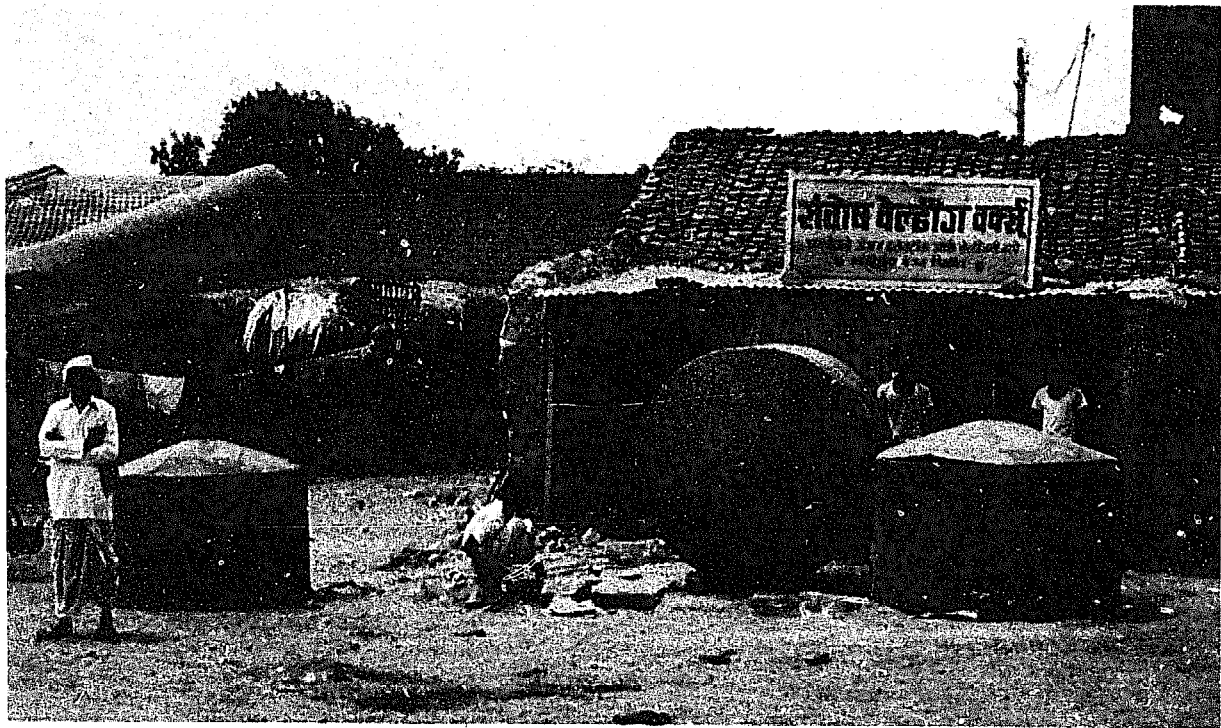
Photo 29: Building metal gasholders in a village workshop in India (Source: Sasse)
