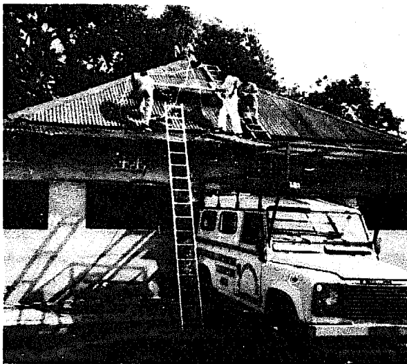
Figure 3.9 Carrying a PV Array onto a Roof
