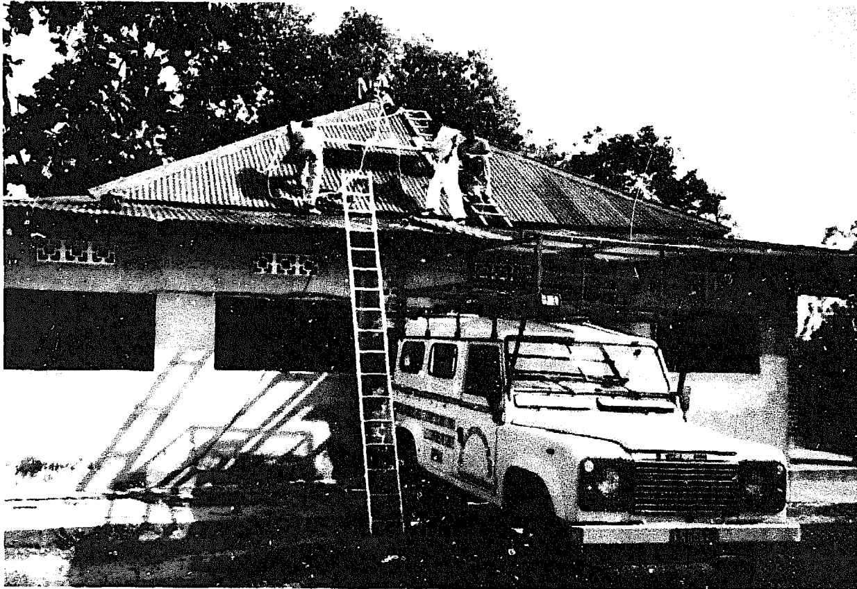
Installing the Solar Array of a Solar Powered Refrigeration and Lighting System for a Health Centre In Zaire (IT Power)
