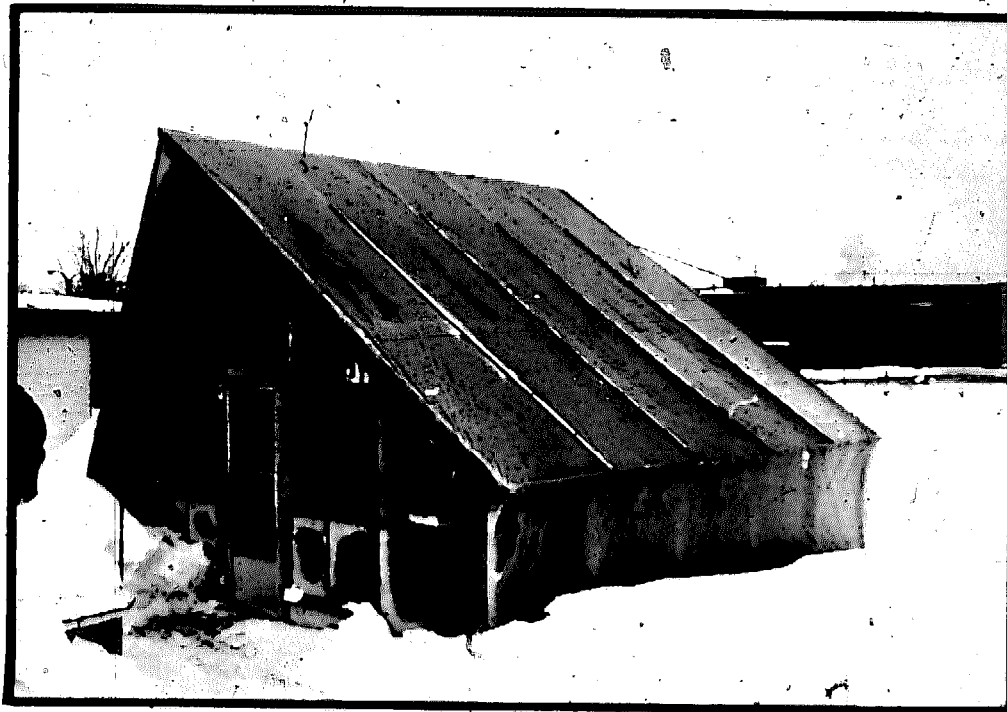
Photo IV-19b: Exterior of Laval University greenhouse. Quebec City, Canada.
