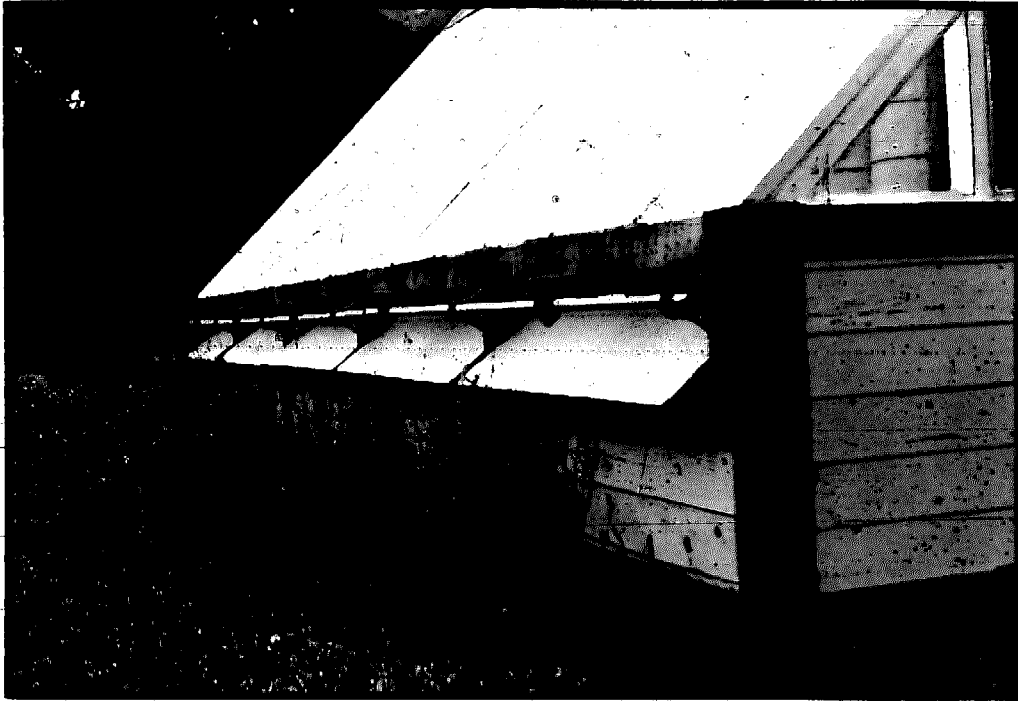
Photo IV-20d: Operable greenhouse vents.
