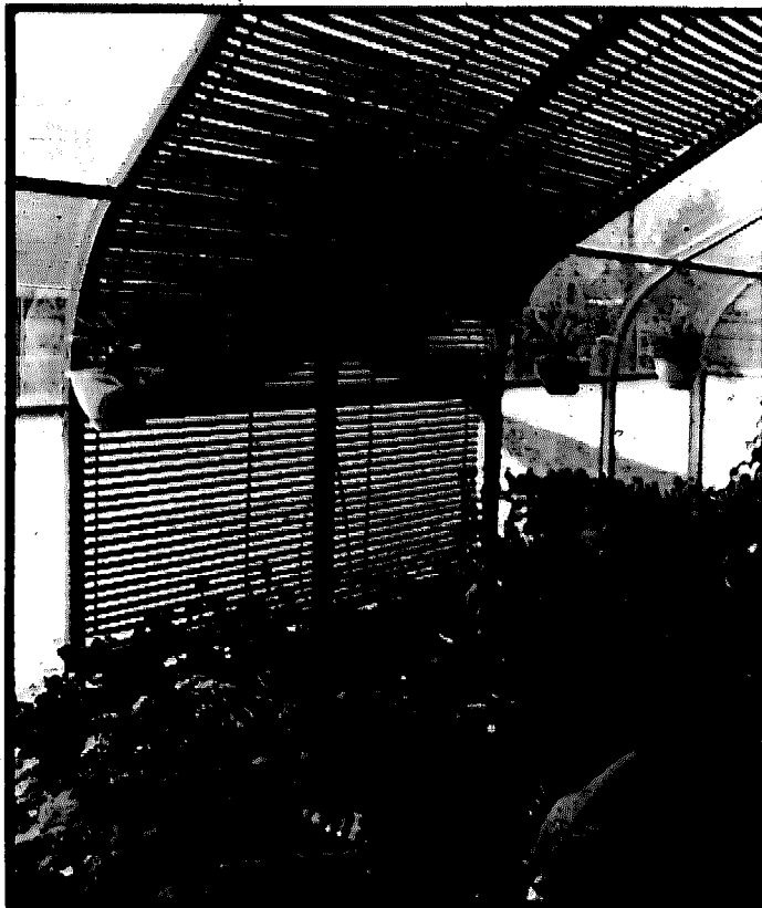
Photo IV-20e: Louvered shading device.
