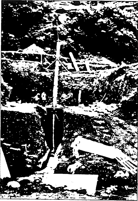
Fig. 29. The penstock, turbine, and draft tube are all assembled and properly aligned before set in concrete. A portion of the tailrace canal has already been completed.
