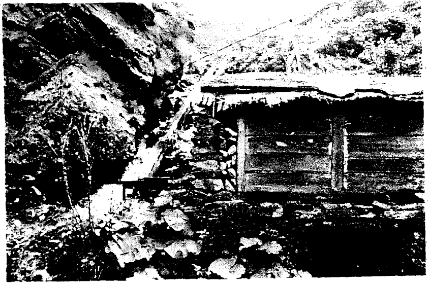
MPPU turbine part at Namche Bazar, at the site of a traditional mill. The square pipe is made of wood. (Project and photo: M.Crawford).
