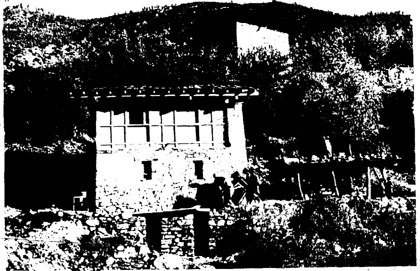
The renovated mill house in Namseling, November 1981. On the left side the upper part of the MPPU, people are transporting the circular saw.
