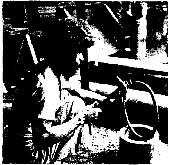
Local manufacture of a low-head pipe flange.
