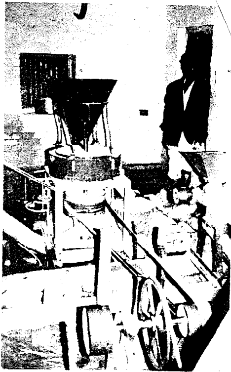
Mill at Thaibo: note the small DC generator attached to the frame.
