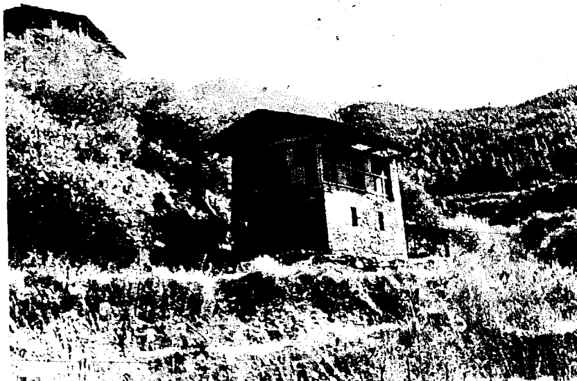
The mill house from the side. On the left side of the house one can see the intake and the pipe. Head = 4 mtr, water flow appr. 100 ltr/sec. With this the MPPU can run the mill, oil expeller and a small dynamo at the same time!
