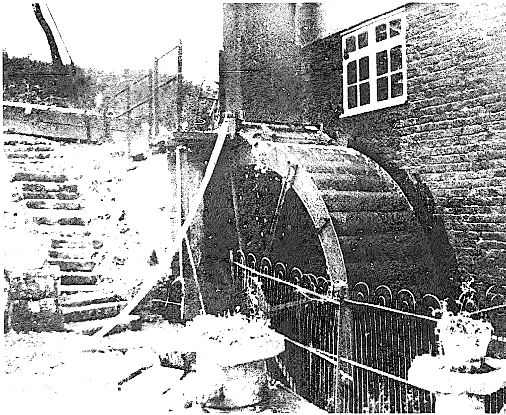
Photo 4 — An old metal water-wheel with head tank giving pressure to the hose
