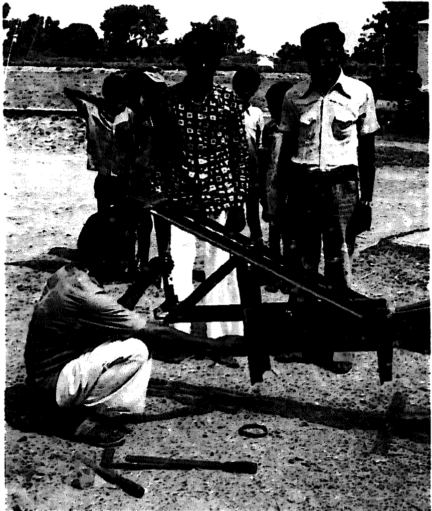
Checking the fit of the head over the tower pipe.
