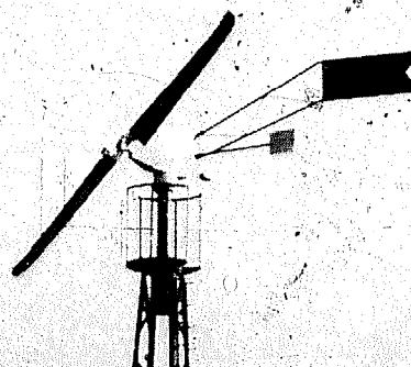
"Ideolec" Wind Generator
