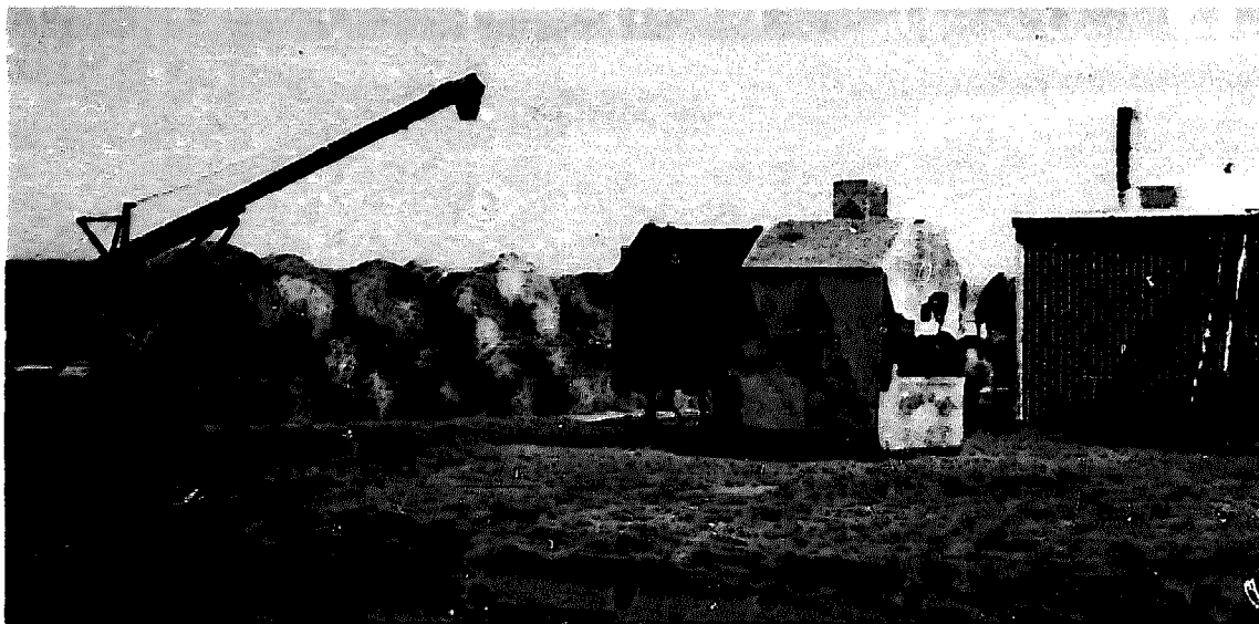
FIGURE 45 Steam boiler designed to operate from rolls of wheat straw (in background).
