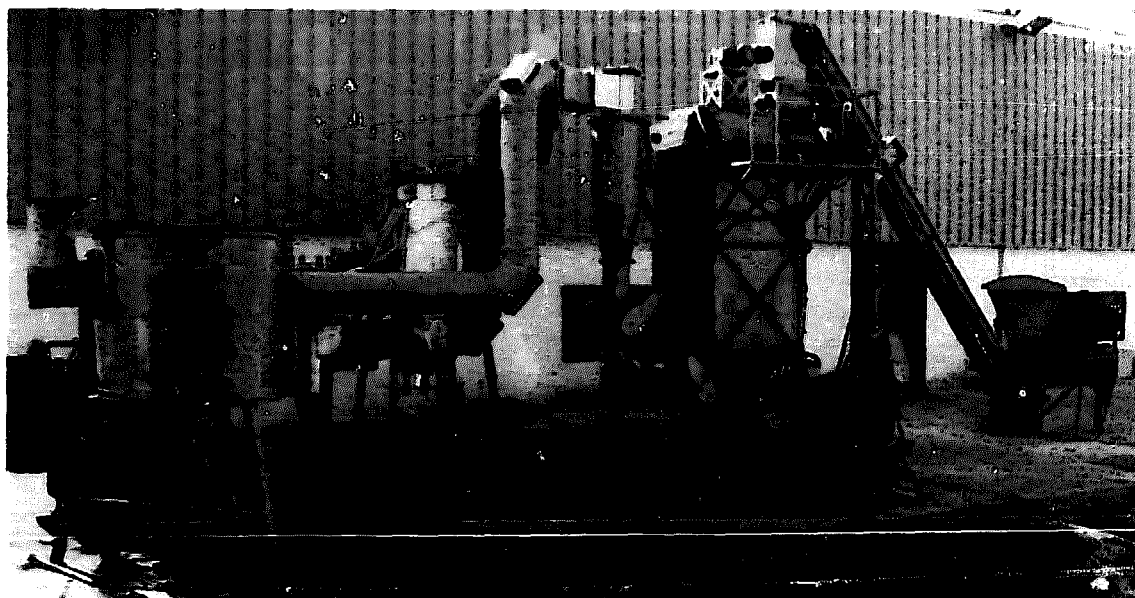
FIGURE 48 A 25-t/day pyrolysis unit developed by the Engineering Experiment Station of the Georgia Institute of Technology.
