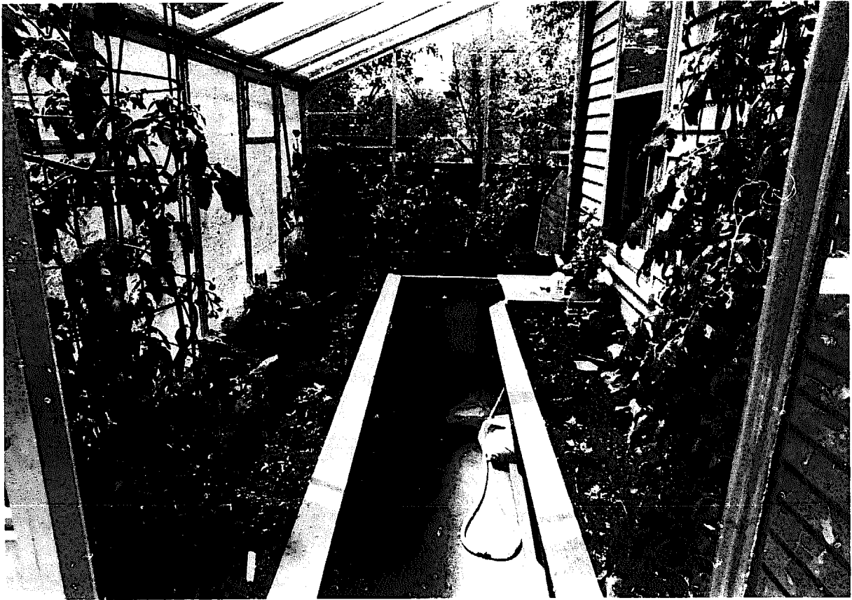
Inside the Cliaus Multum experimental solar greenhouse. Note the deep planting beds through which the greywater is filtered.
