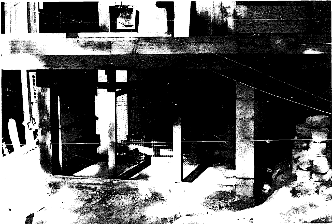
This photo of the unfinished retrofitted privy shows the heavy wire mesh separating the composting bin from the two storage bins. (Photo by Susie Benson.)
