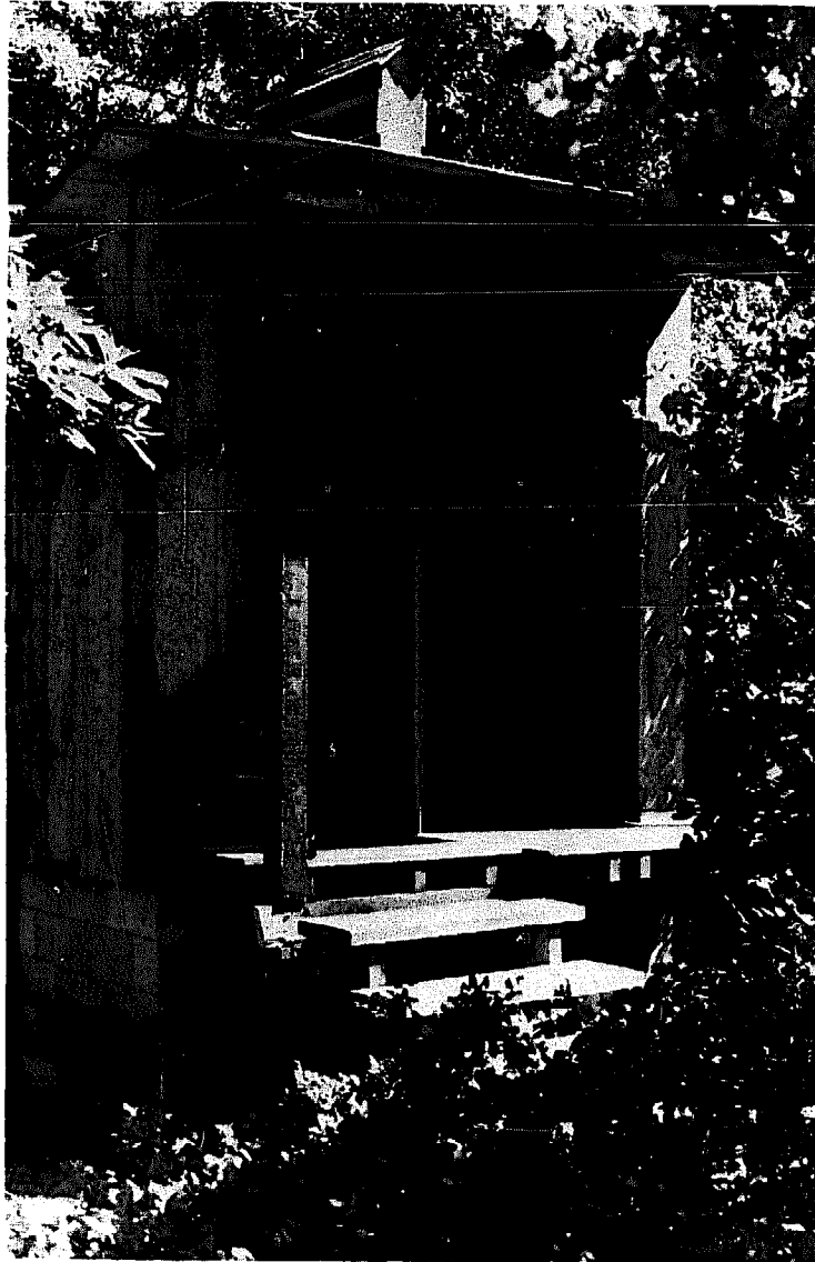
Front view of the modified two-holer at the Farallones Institute's Rural Center. (Photo by Peter Webster.)
