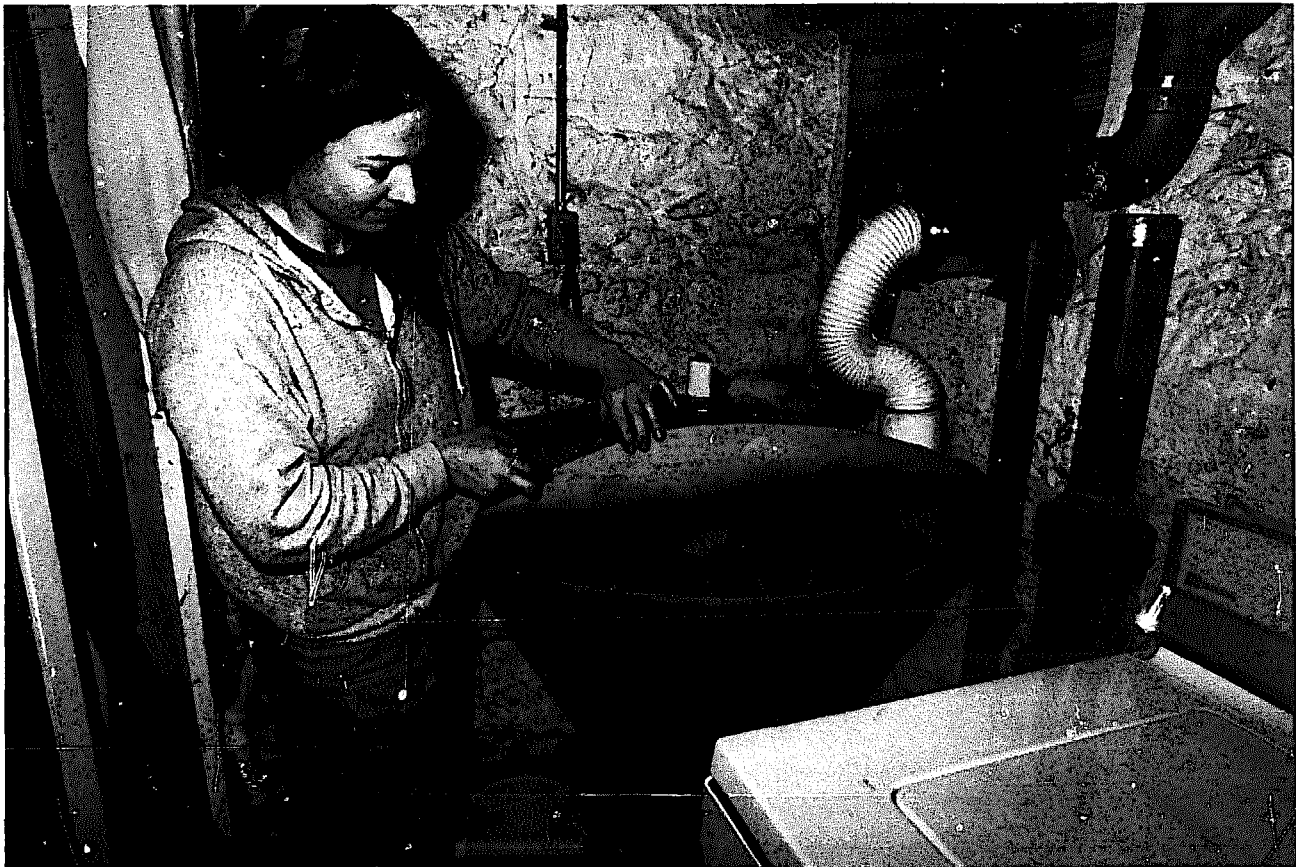
Abby Rockefeller lifting up the cover on the trickle filter, the first stage in her greywater treatment and disposal setup. At right, note how water pipe from sinks and laundry was diverted from sewer hookup to trickle filter.
