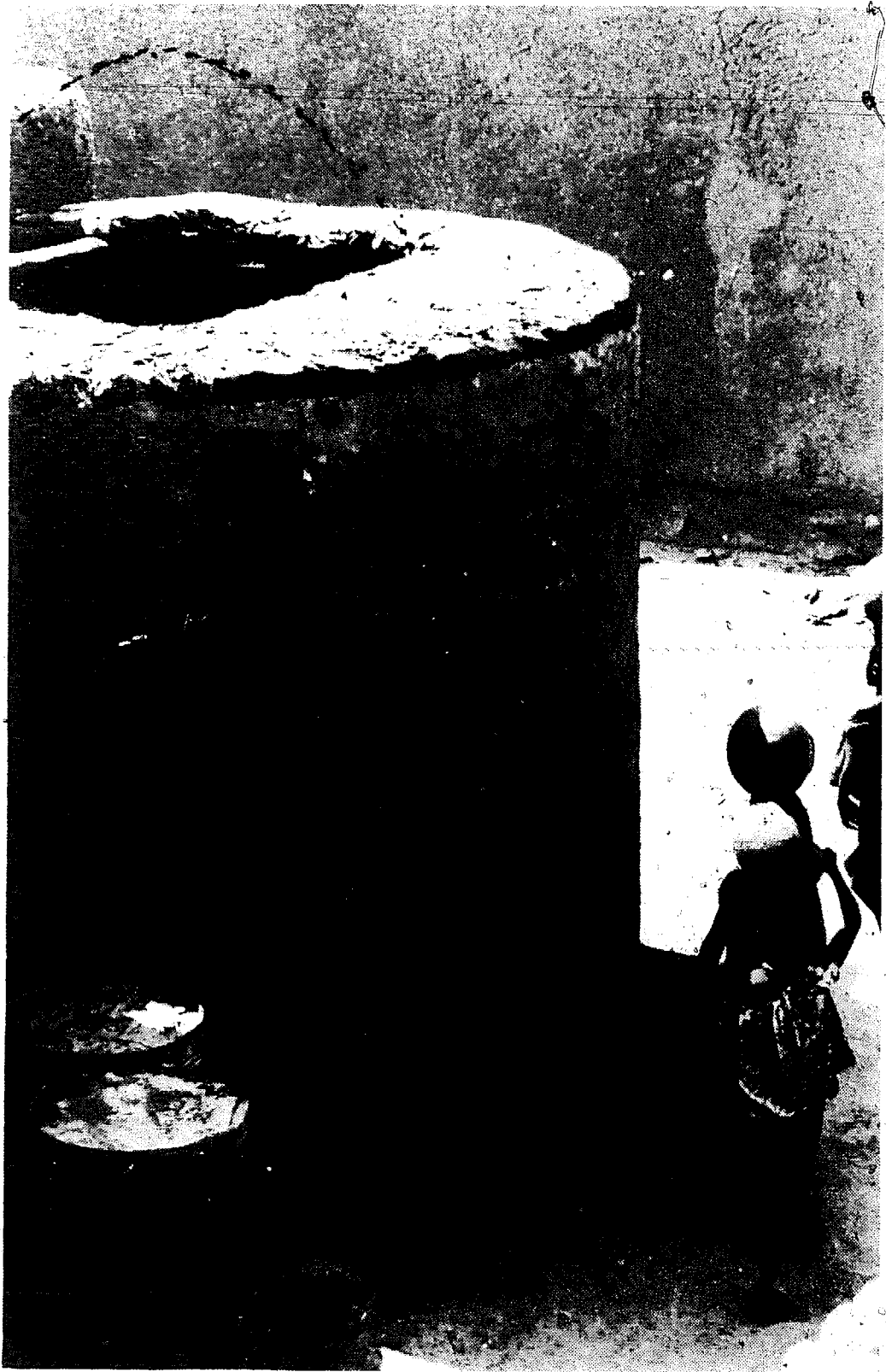
Photo 6 Ferrocement-lined adobe granary bin under construction. Mali
