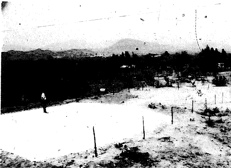
9.9 Catchment area for tank with wire fence.
