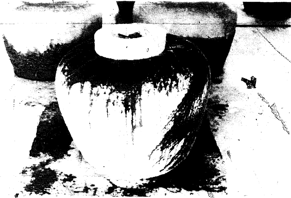
2.7 Place a circular ring on the top of the sack to make a mould for the opening of the jar. This can be made of wood or precast mortar.
