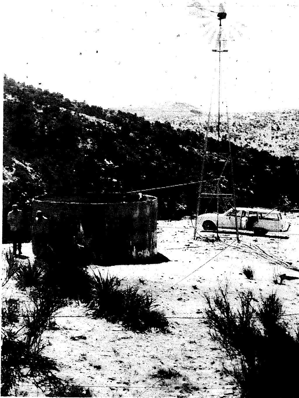
10.5 Water pumping into tank
