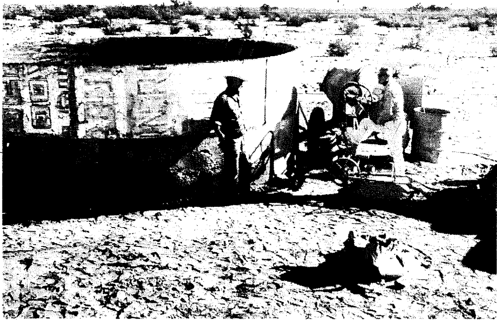
10.1 Cheap shuttering from flattened oil drums
