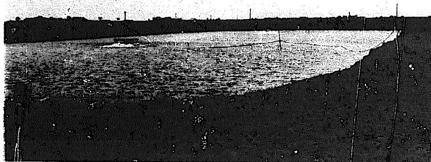
Fig. 22 Floating aerator as used at the Jie-fang People's Commune, Shanghai
