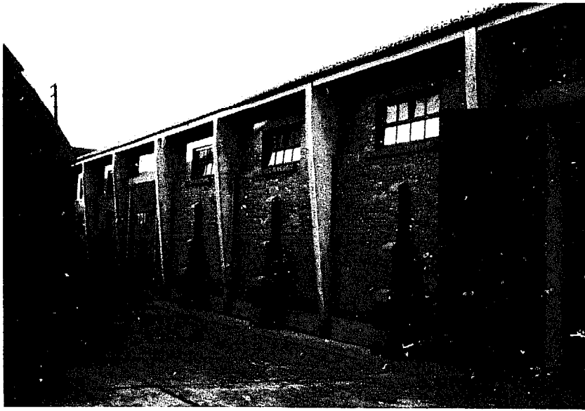
Photo 49 - Warehouse for bagged grain. Portal frames at cc 4 m. Buttresses between portal frames. (Seventh Depot, Shanghai)
