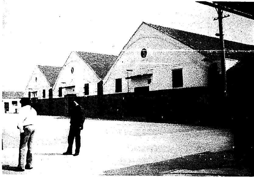
Photo 45 - Concrete dome-roofed warehouse with tile roof. Three bays, each 16 x 20 m. Built 1959. Total holding capacity 1 500 tons paddy. (Bacon Depot)
