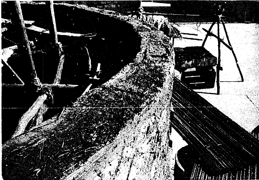
Photo 29 - 20 cm thick silo wall. Density of the clay/straw wall must be 966 \text{ g/cm}^3 or more.
