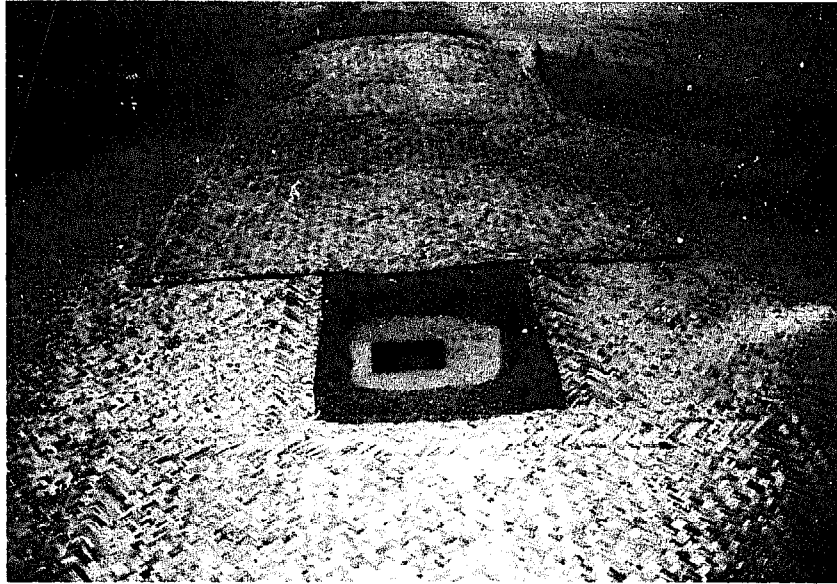
Photo 8 - Fibre mats on the floor of a clay/straw silo (South Gate Depot, Songjiang County, Shanghai)
