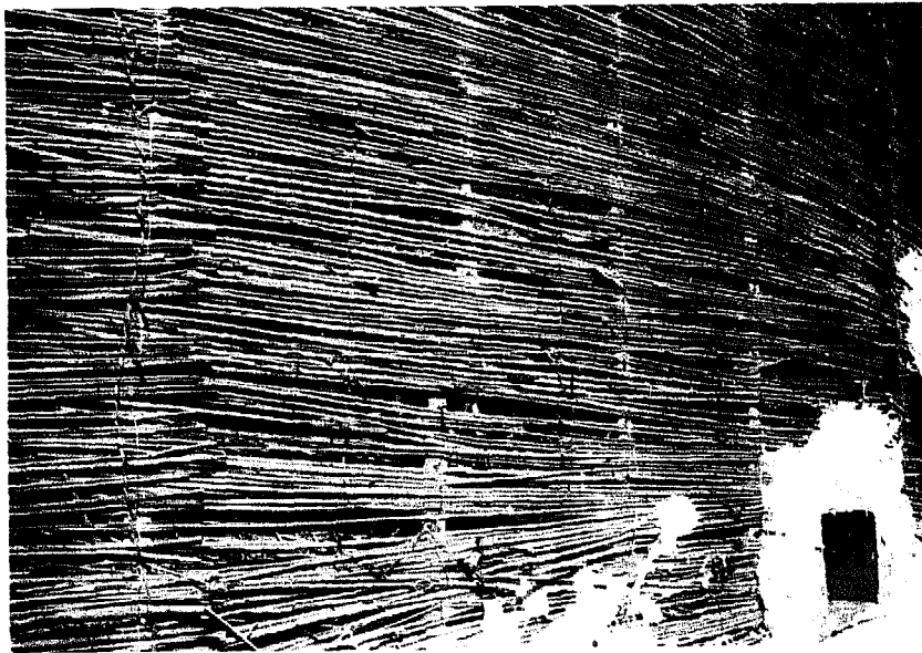
Photo 35 - Waterproofing of silo wall. Reed mats fixed on wooden laths. (Niou Pao Tun Depot)
