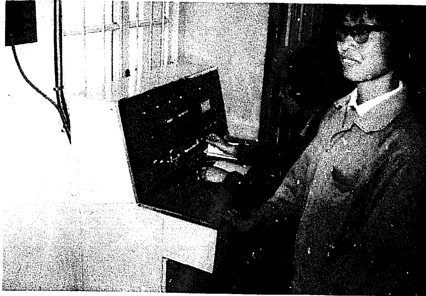
Photo 14 - Central temperature registering panel (Baoan Depot)
