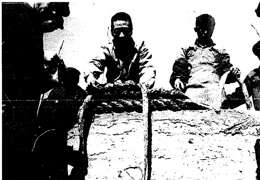
Photo 33 - Third layer of eaves. The top surface must be kept level by placing clay/straw bundles along the wall. (Niou Pao Tun Depot)
