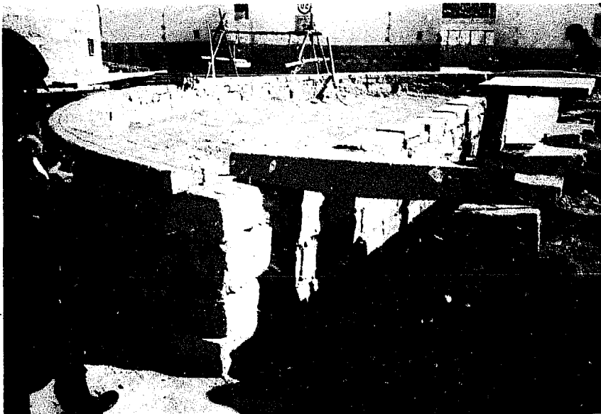
Photo 21 - Stone foundation with two layers of brick. Central channel for mechanical removal of grain. Covered by prefabricated concrete slabs. (Niou Pao Tun Depot)
