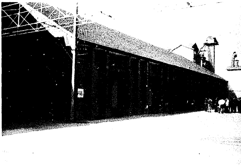
Photo 40 - Bulk grain warehouse, two sections, 20 x 24.5 m each. Type "51". (First Depot, Wuxi)
