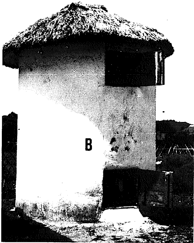
Figure 21. Simple, small rustic stores with outside painted white. A -- Timber construction, 1.5 TM capacity (CIP, Huancayo, Peru). B -- Lath and plaster and mud brick construction, 2 TM capacity (Mountain State Agricultural College, Baguio, Philippines).
