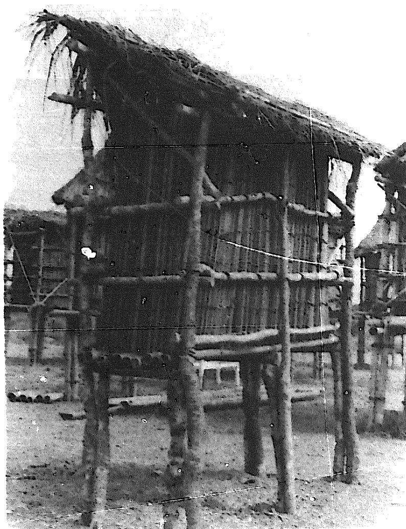
Crib constructed entirely from local materials (Courtesy W. Boshoff)
