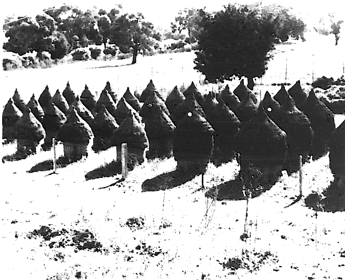
Traditional mud-walled stores of the low savannah zones, West Africa (Courtesy W. Boshoff)
