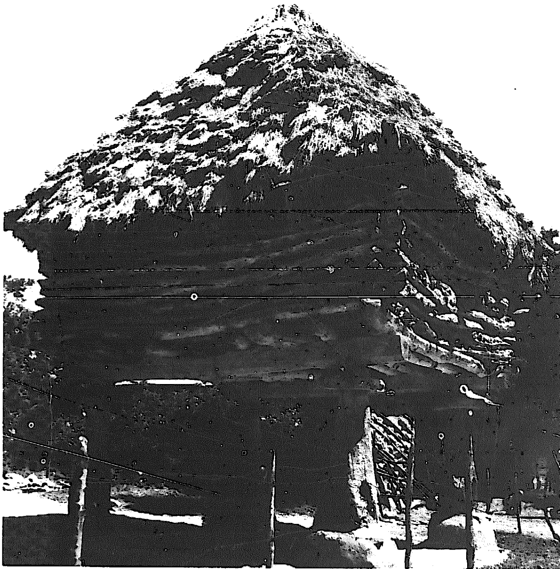
“Kanduch” lath and clay rice store, Chasemabad District, Gilan Province, Iran. Note the log-disc rodent baffles. (FAO photo)
