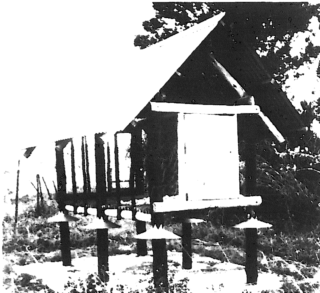
TP1 Recommended mesh-sided crib, Swaziland. Note the corrugated iron roof and metal rat guards. (Crown copyright, Courtesy TPI)
