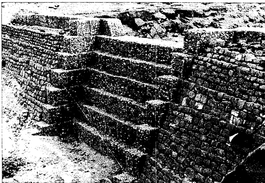
Weir made from gabions and dry-stone work (Cape Verde)
