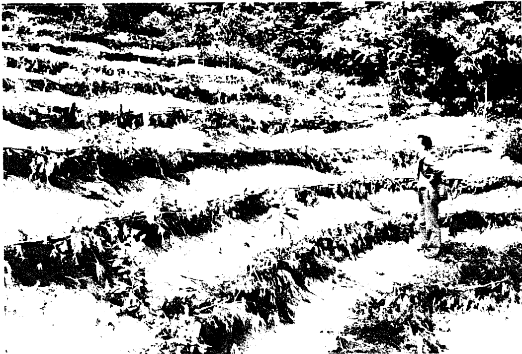
Figure 3. For comparison sake , an example of the somewhat different style of wattling and staking ("clayonnage") more commonly known in the European countries. (Photo: U.S. Forest Service)
