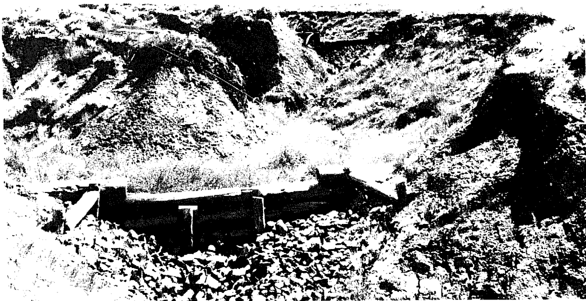
Figure 4. Conservation measures often may rely on local materials and hand labour, for example, in gully correction work with small logs and rocks (Photo courtesy of U.S. Forest Service).
