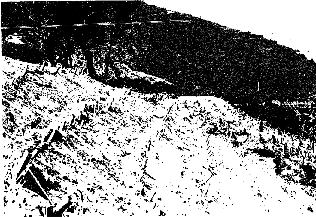
Figure 2. Wattling and staking done under the special Employment Programme along a forest road, Mt. James Forest District, Jamaica, 1975 (Photograph made by the author shortly after work completed)
