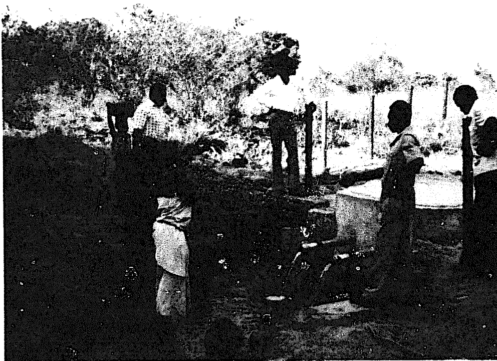
Spring protection, Soroti District, Uganda (Stern).
