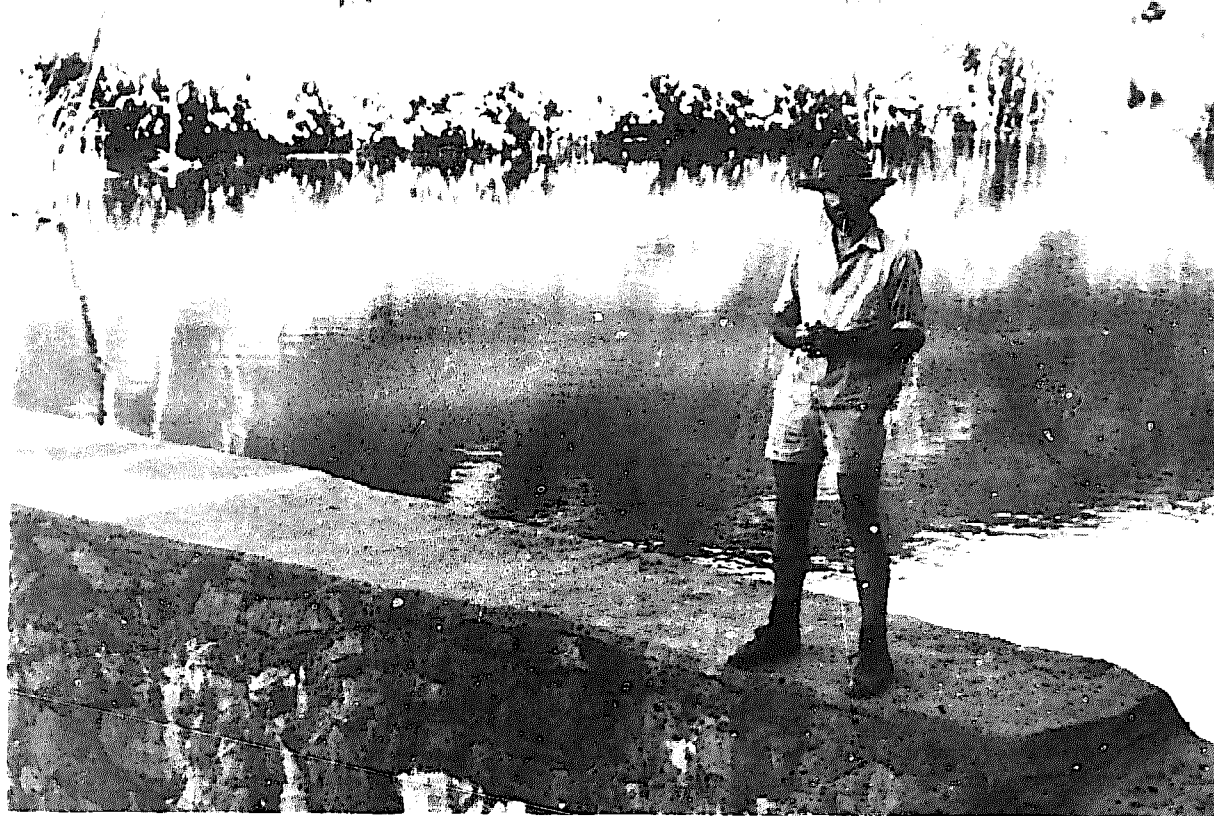
ALLEN JENKINS AT ULLUMPARA DAM IN A ROCK-WALLED VALLEY. DAM PLATE 5-5 PROVIDES AMPLE GARDEN WATER AT HEAD. MANY SUCH SITES ARE AVAILABLE IN DESERTS.
