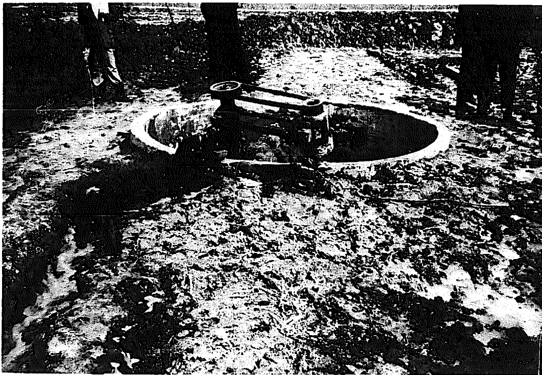
Fig. 46 Outlet of large size bio-gas plant. Effluent pumped into irrigation drain. Cheng Hsiang Production Brigade, Jiangsu Province.
