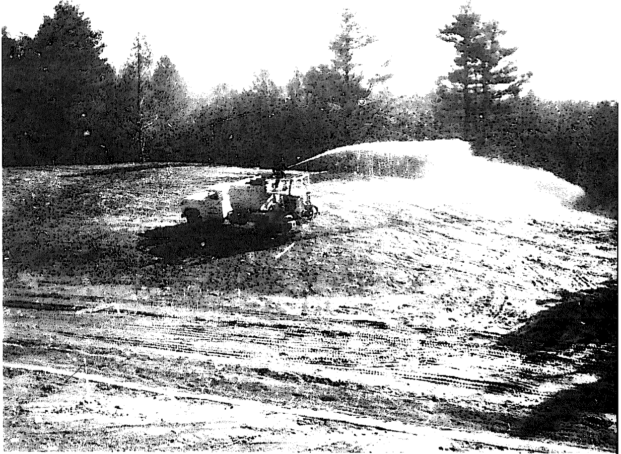
Fig. 13-11. Hydroseeder spraying a water solution containing seed and fertilizer on newly graded slope.
