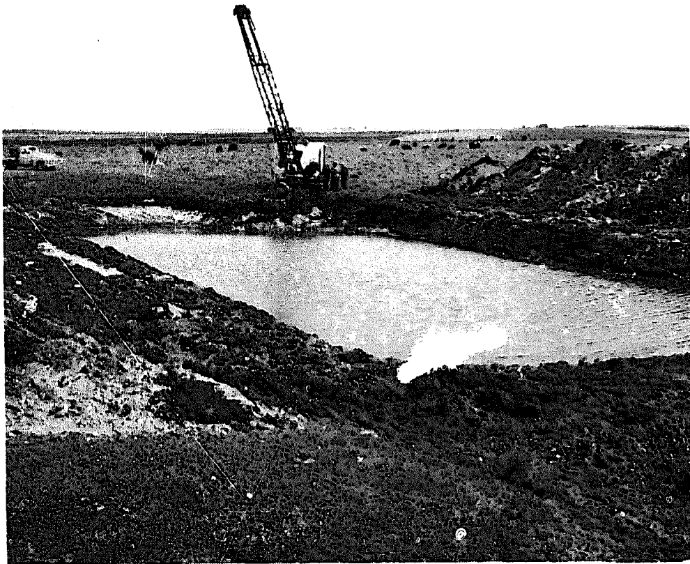
Fig. 11-17. Excavating a pond with a dragline.
