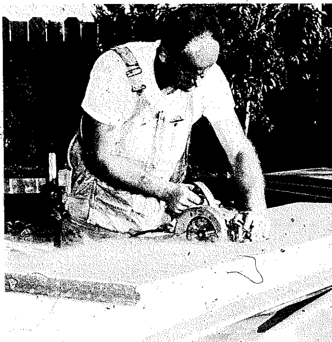
On soft materials like this roof-deck insulation, you can make a maximum cut on one surface and then snap the material to break uncut section. If appearance of the cut is important, then, of course, you must cut from both sides.
