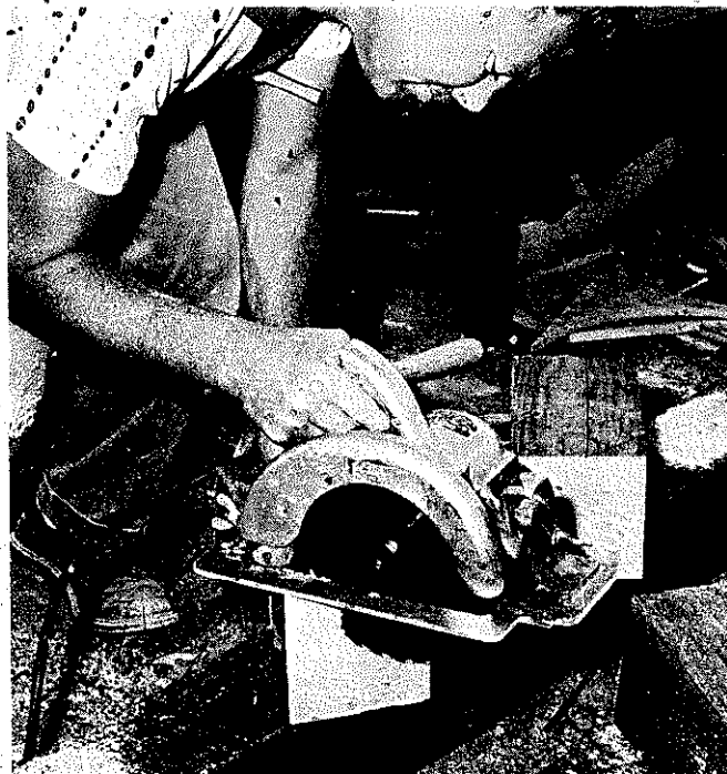
You can get through extra-thick stock by making matching cuts from opposite sides. Good layout and accurate placement of the saw for each cut are important.
