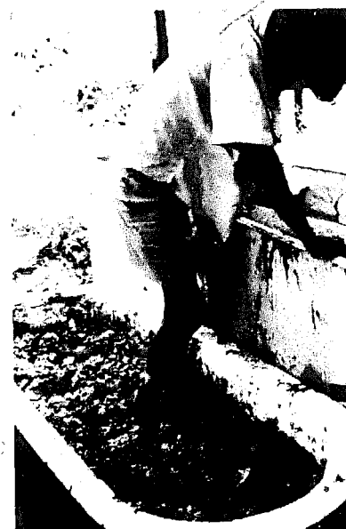
Trampling clay for the furnace lining, Ghana.
