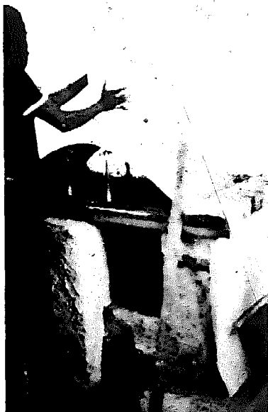
A melt-out furnace in the course of construction, Ghana.
