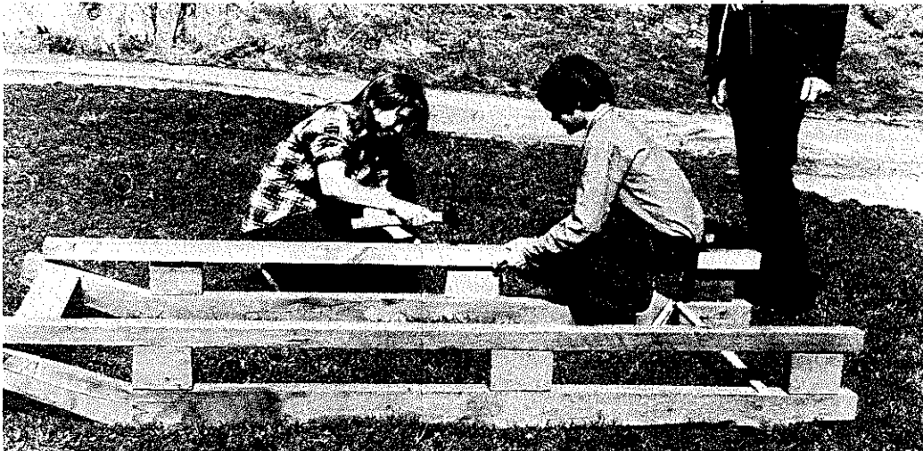
PLATE 167 Now the hemlock sills are tacked into place. They will be set permanently later. They hold the floor of the sled up off the ground so that it can be pulled over rocks and stumps without hanging up.
