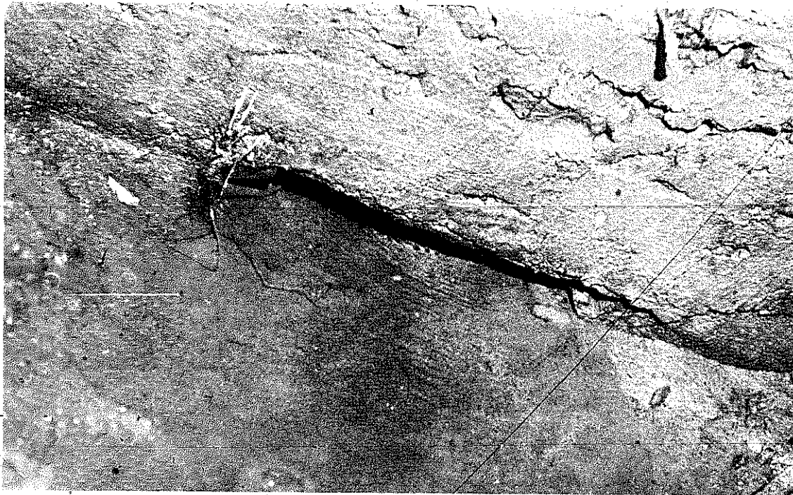
PLATE 321 Point D, view of water coming under a small partition as it goes through the trough.
