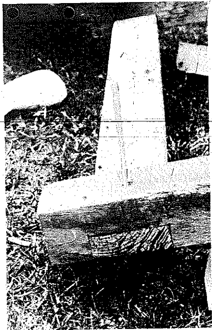
PLATE 170 When the wedge is in place, as shown here, again a saw is used to cut it off flush with the bottom of the runner.
