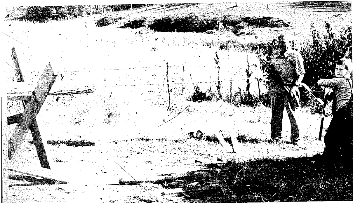
PLATE 310 Garnett begins to bore out the log as his grandson looks on.
