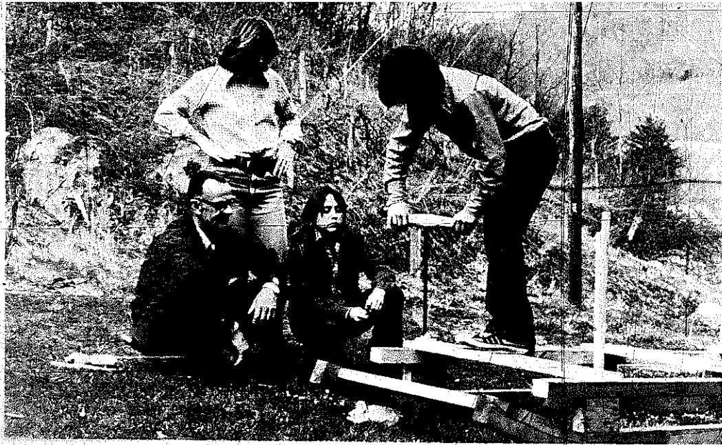
PLATE 172 With the 1" auger, Dwayne drills down through the oak crosspieces, the sills, blocks, and well into the runners. Long dowels driven into each of the six holes hold the sled together and keep such loads as logs from rolling off.
