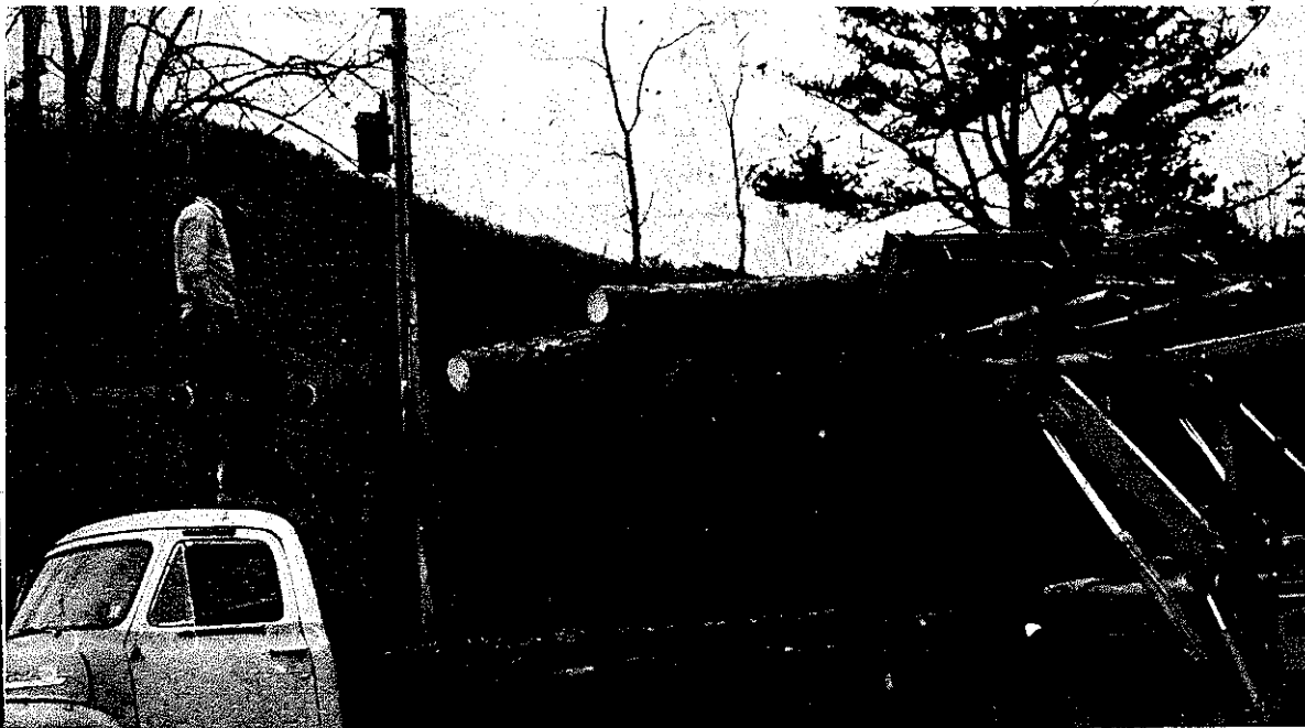
PLATE 281 Truck being unloaded after passing under the saw.
