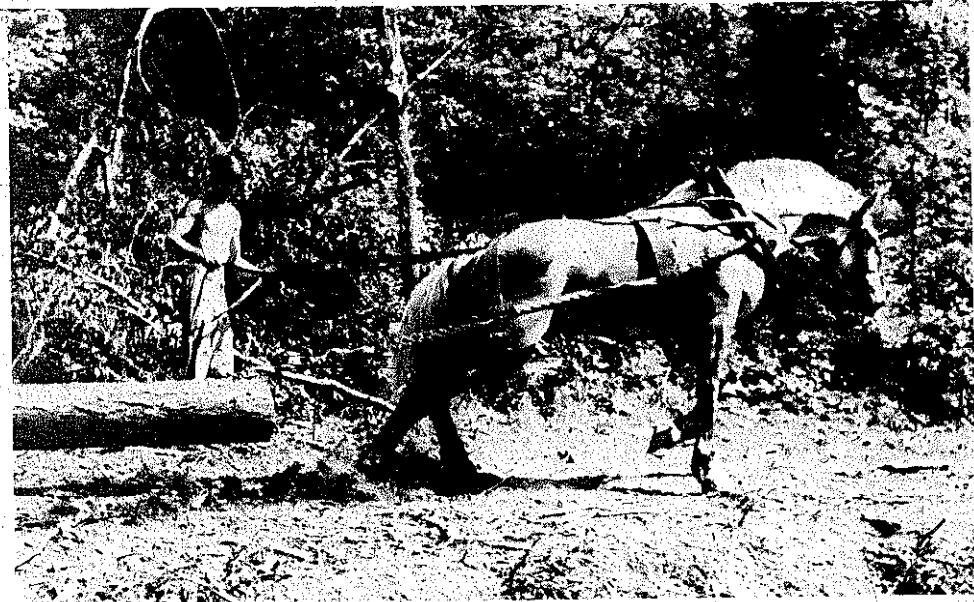
PLATE 266. When the logs are hooked together, Millard's horse, Charley, is backed up to the lead log and chained to it via the singletree at the end of his harness, and a "J-grab" or "header grab" that connects the singletree to the lead log. At a signal from Jack, Millard's son, Charley lunges forward to get the train of logs moving.
