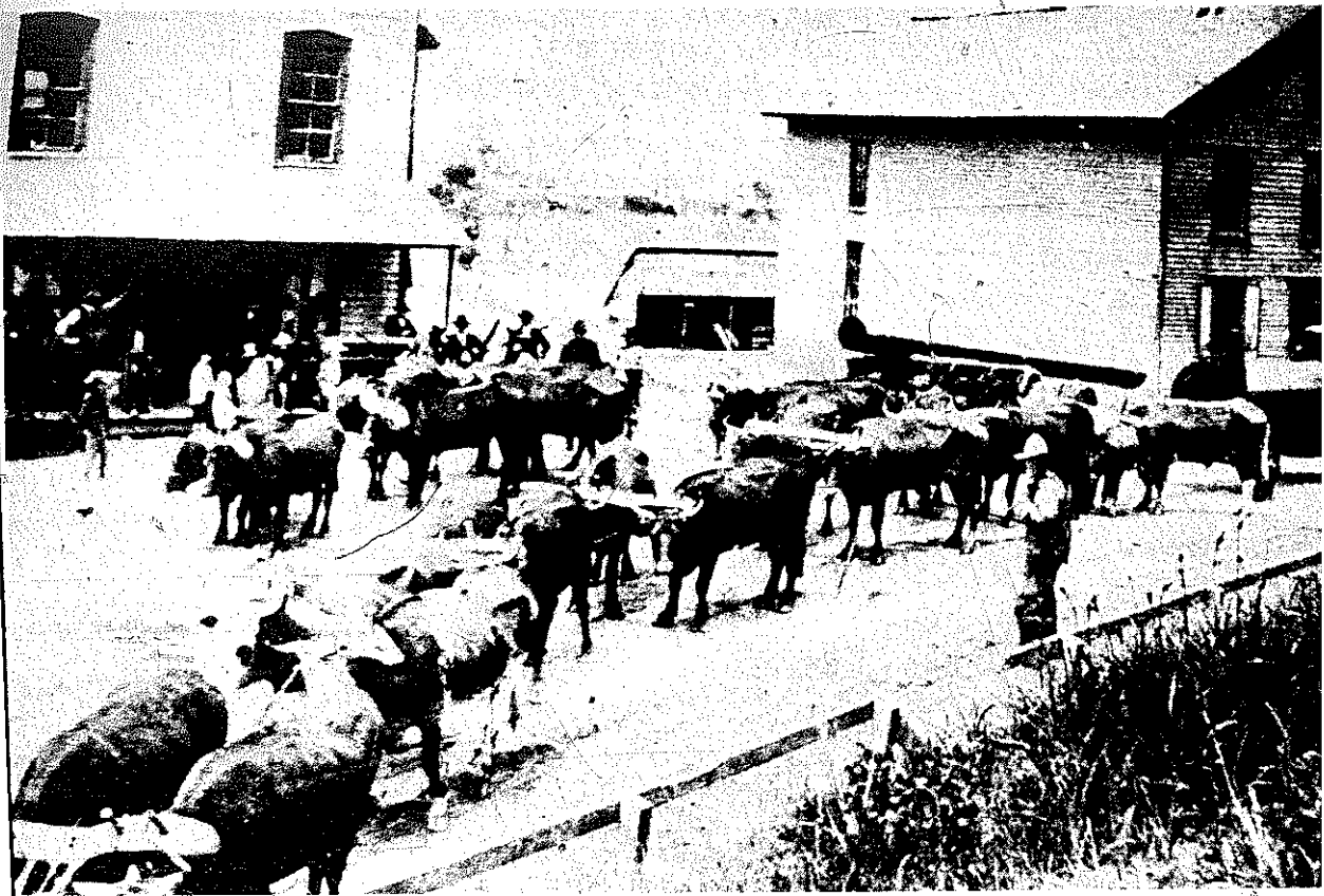
PLATE 279 Bud Allen or Suel Medford moving a steam sawmill. Eight pairs of oxen (one pair is not visible beyond the lower left corner) are hitched to the boiler (far right), and four more pairs behind them are hitched to the long stack and saw box. This scene was probably photographed in the Pigeon Valley. (Photo courtesy of Champion Paper.)
