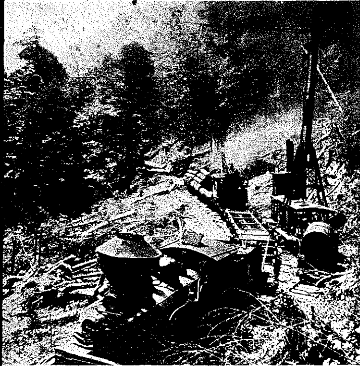
PLATE 277 At the head of the railroad line, an overhead skidder (far right) powered by a steam boiler would be used to drag the logs out of the woods, where they had been cut, to the loading area. There a log loader (or "stiff-necked loader"), visible in this photograph on the tracks beyond the steam engine, would load the logs onto the railroad cars for the trip to the mill. When one car was filled, the loader would pull off the main track onto a short siding so that the engineer of the train could move another empty car into position to be loaded. (Photo courtesy of Champion Paper.)
