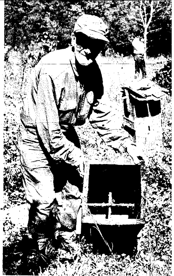
PLATES 13-15 Lon Reid's plank gums are the next step in the evolution from hollow tree trunks to modern supers. Lon's gums also have the wooden eyes for holding the heads on tightly (13), and the crossed stick design (14). To make sure the lids stay on, Lon piles rocks on most of them (15).
