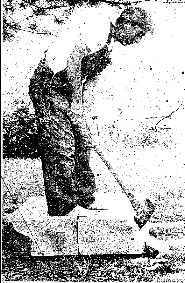
PLATE 137 With an axe, he hews the wheel out round.
