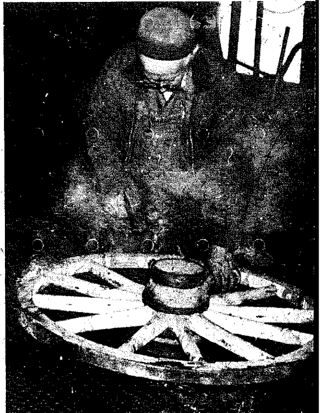
PLATE 114 As the wood smokes from the heat, he pounds the tire down evenly all the way around and douses it repeatedly with water to finish the job.
