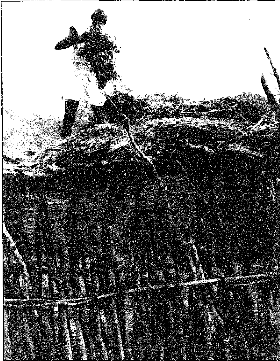
Model of local shelter for oxen, with stocking of fodder from above.
