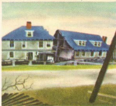
Waves undermine buildings.
