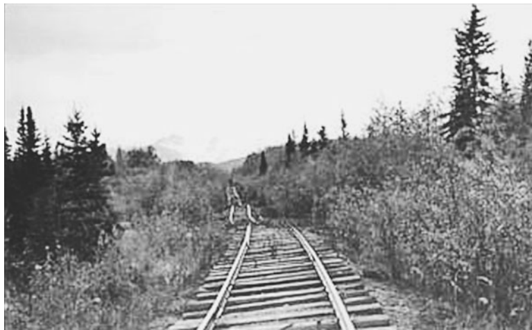
Figure 3-19 Copper River and Northwestern Railway track built on Alaska permafrost. (Source: NASA; credit: United State Geologic Survey.)
