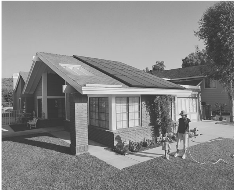
Figure 8-6 Roof-mounted photovoltaic system. In many locations, utility companies purchase solar-generated electrical power from customers. (Courtesy: BP Solar.)
