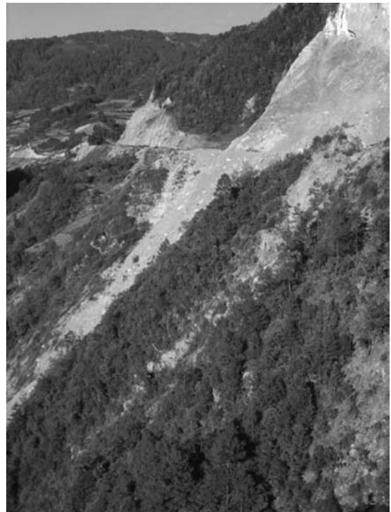
FIGURE 12.8. Epic levels of landslide erosion along the newly constructed Weixi–Shangri-La road in Yunnan, China.
