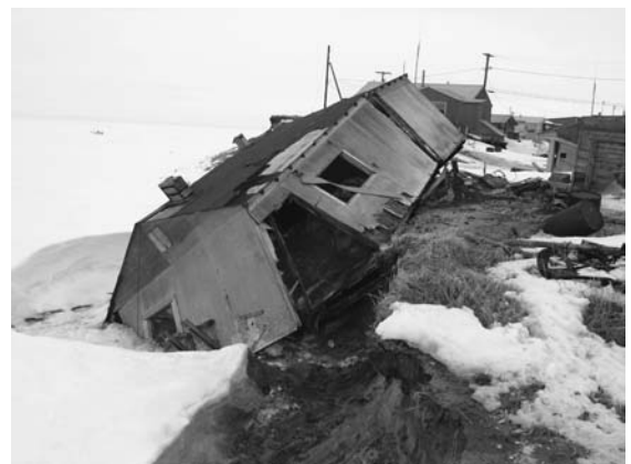
FIGURE 13.8. Shishmaref, an Alaskan village severely affected by coastal erosion, April 2007 (photo by D. Fortier).
