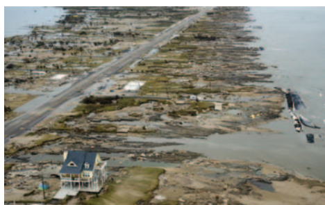
PLATE 48. The community of Gilchrist, Texas, on the Bolivar Peninsula between eastern Galveston Bay and the Gulf of Mexico, was almost totally destroyed by the US landfall of Hurricane Ike on 13 September 2008. The geomorphological damage has been described as landscape 'scarring', affecting over 400 km of the Gulf coastline (photograph: David J. Phillip – Pool/Getty Images).
