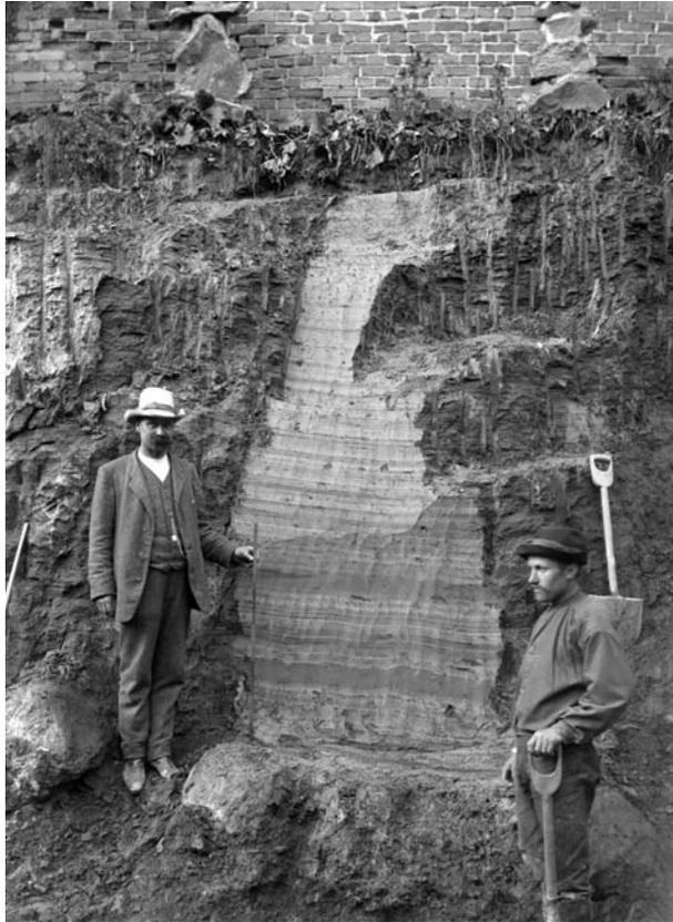
**Figure V1** Varved glacial clays in Tampere, southern Finland, which were deposited in the early Holocene Baltic basin. (Photo by J. J. Sederholm, 1907.)
