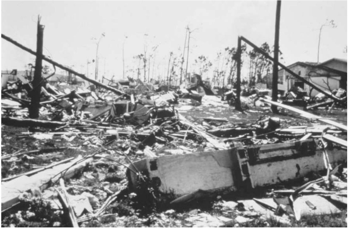
Plate 22 Ground view of the devastation caused by Hurricane Andrew in Pinewoods Villa, southern Florida, 23–24 August 1992 (courtesy of NOAA, NOAA Photo Library Historic NWS Collection wea 00534).
