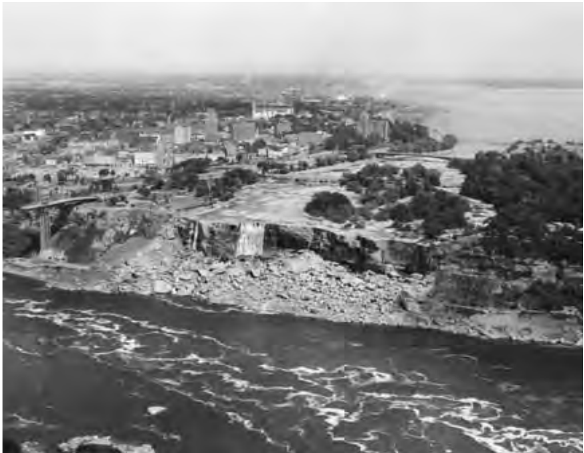
Vast amounts of talus lie exposed in this historic photo from June 1969, when engineers dammed water flowing toward the American Falls at Niagara Falls. (Ron Roels)
