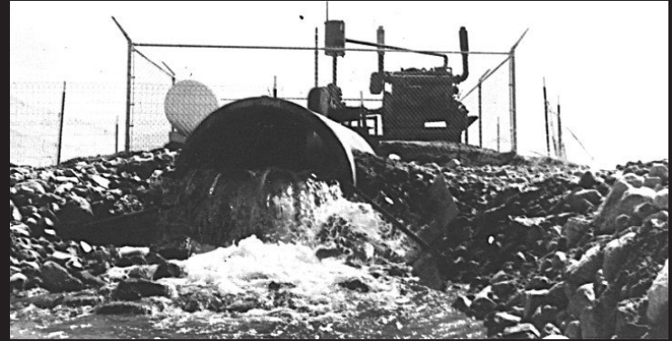
The first Lake Elsinore well tested a consistent flow of 5,500 gallons per minute from a deep seated primary water source.
