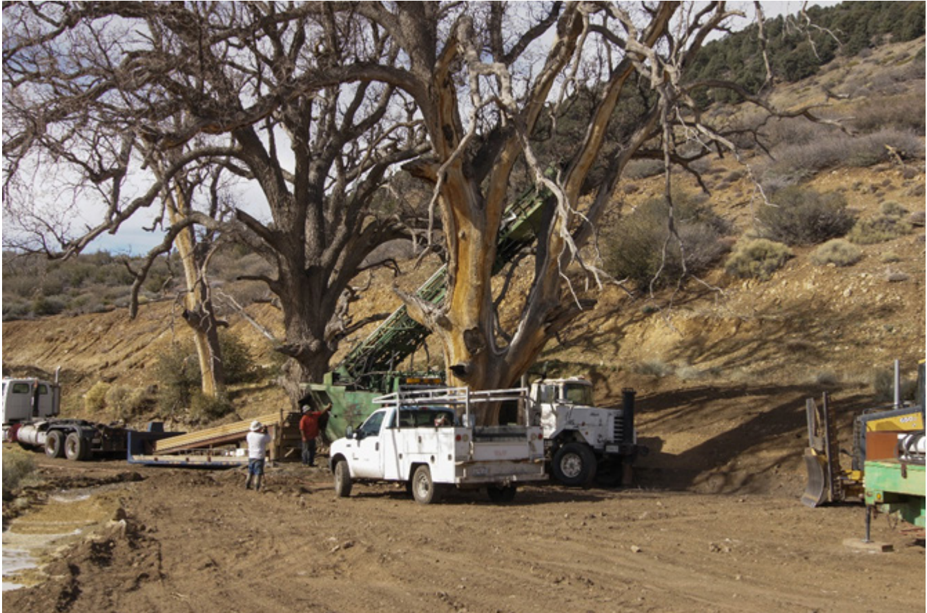
Note: the presence of two ancient large oaks at location. The trees were an indicator of the presence of water.
