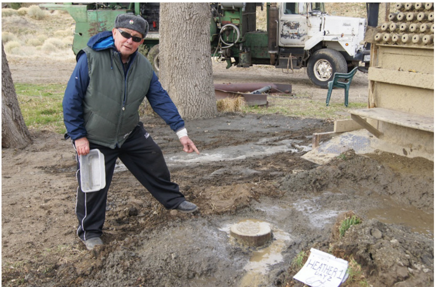
Pal points to artesian water which surfaced from the borehole.
