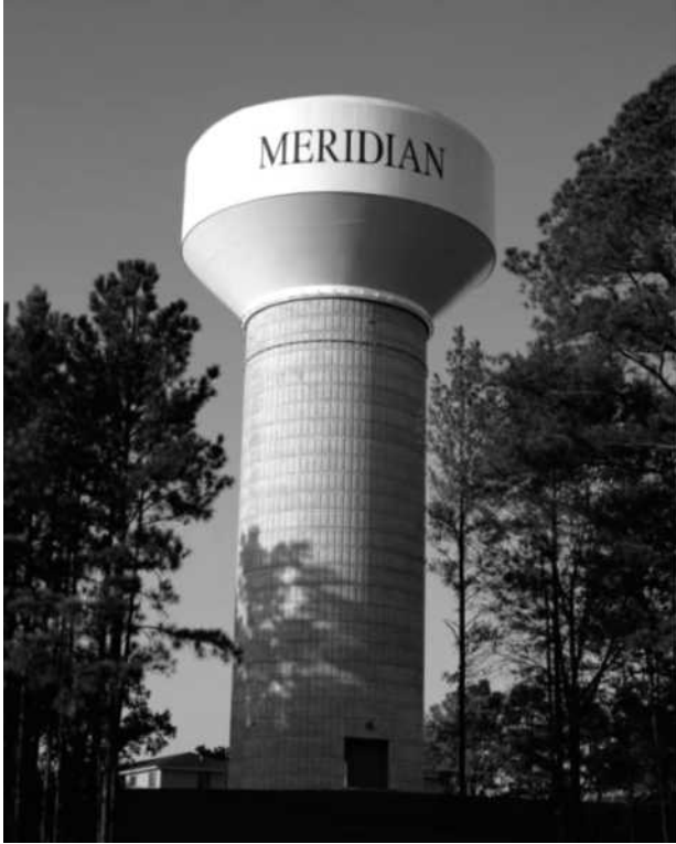
Figure 3. Composite elevated storage tank (Source: Caldwell Tank, Inc.).
