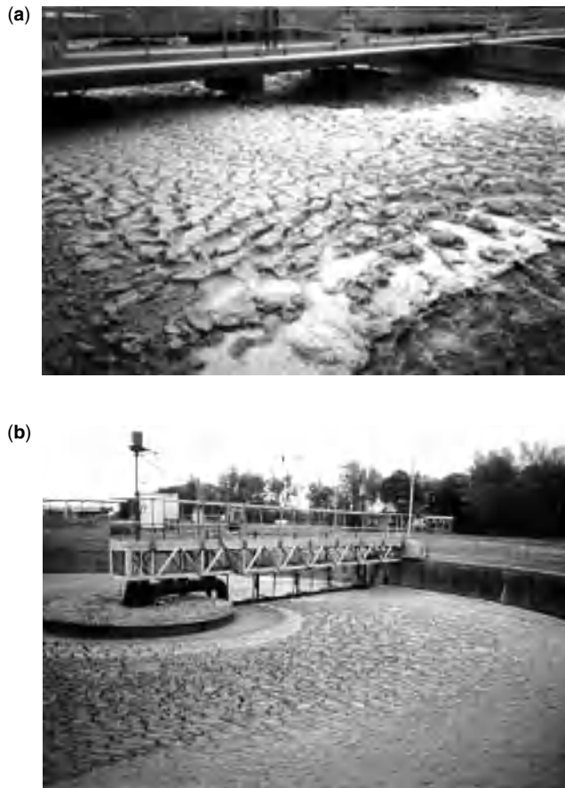
Figure 1. Microbial foam on the surface of (a) a mechanically agitated aeration basin and (b) a final clarifier, where it has partially dried out placing the tank out of operation.
