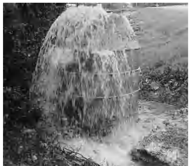
Overflowing sewer due to a sewer blockage
