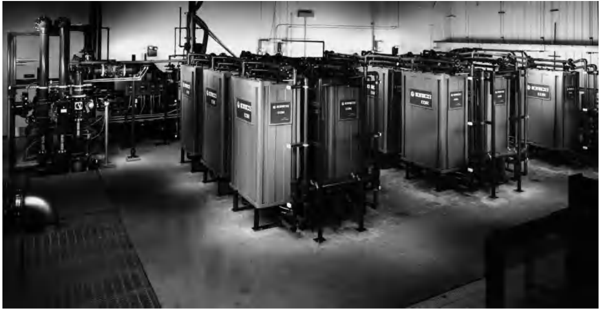
Figure 4. San Diego took a major step in the late 1990s by equipping a new high-technology wastewater reclamation plant with EDR (electrodialysis reversal) system from Ionics, Incorporated, to desalinate tertiary treated wastewater.
