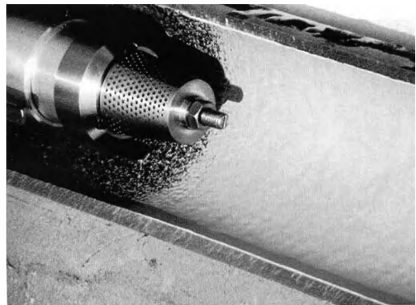
Figure 6. Application of epoxy resin lining.
