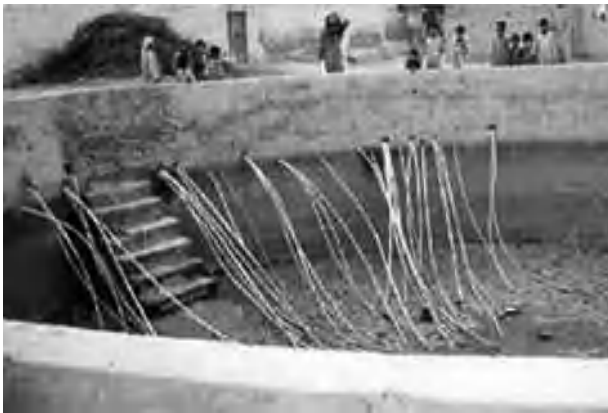
Figure 6. House connections in dry tank.
