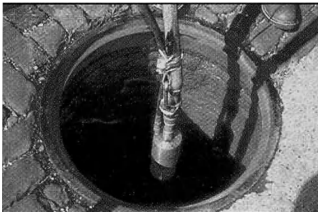
Figure 8. Application of one-coat cementitious structural liner.
