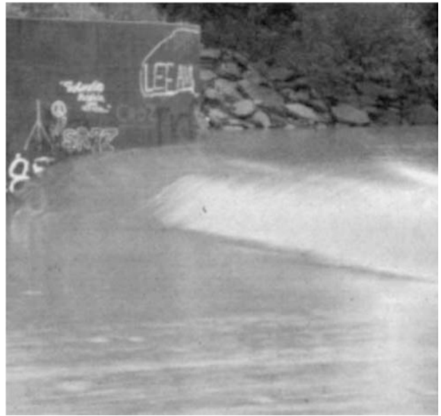
Fig. 6 Smooth flow over ogee spillway crest.
