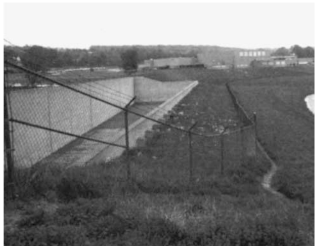
Fig. 4 Side-channel spillway.
