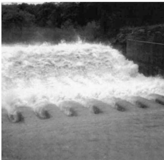
Fig. 9 Energy dissipation basin.
