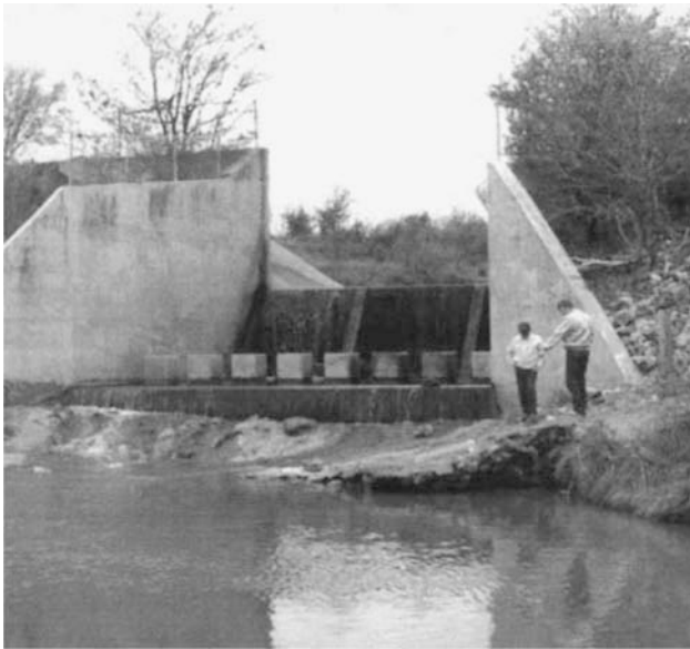
Fig. 1 Straight-drop spillway.
