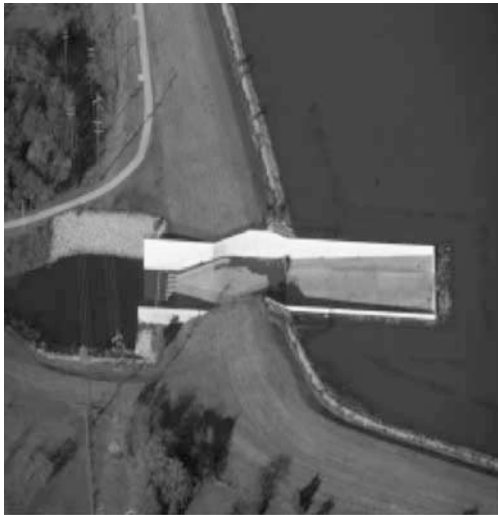
Fig. 7 Chute spillway with notched box inlet.
