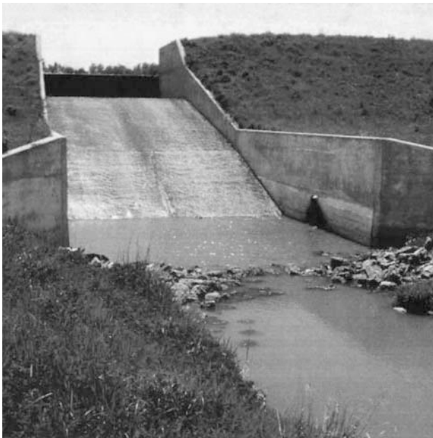
Fig. 2 Chute spillway.
