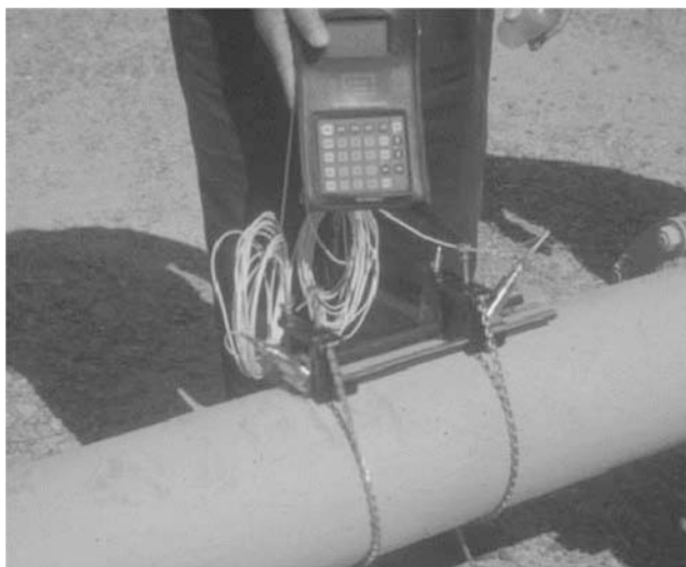
Fig. 3 Portable ultrasonic flow meter on outlet pipe of an irrigation well. Sensors are usually mounted on the side of pipe to avoid air bubbles that may be in the pipe.
