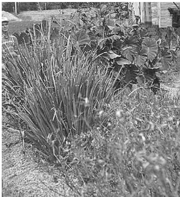
Fig. 4 VSB wetland for treating onsite residential wastewater. This system uses gravel media and variety of wetland plants. (Photo: Barbara Dallemand.)
