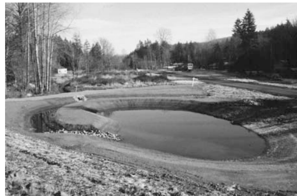
Fig. 2 Detention pond serving a residential development and constructed to a peak discharge standard in the late 1980s, King County, Washington. Inlet channel functions as bioswale (visible at left); outlet drains under road to right.
