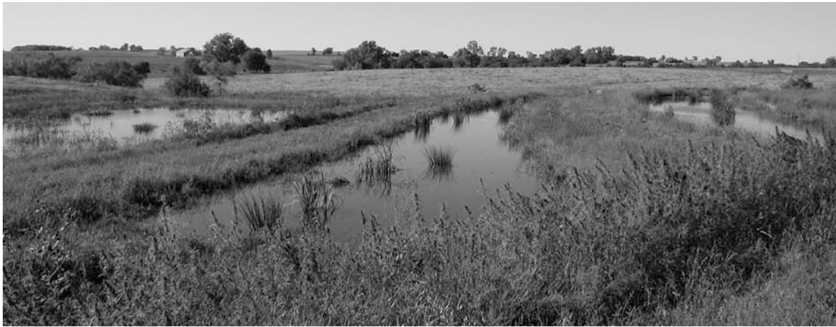
Fig. 2 A three-cell, FWS wetland for treating dairy wastewater. This system is in its first year of operation; plants were recently established. (Photo: Peter Clark.)
