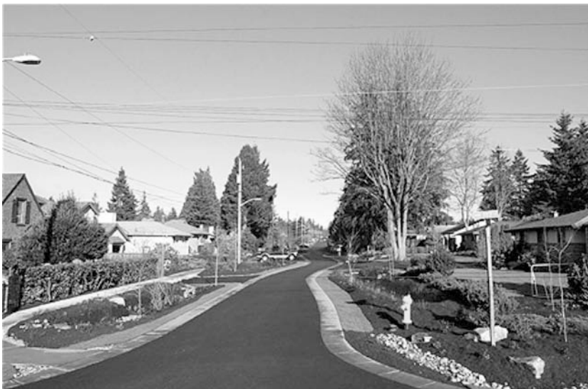
Fig. 2 Retrofitted residential block in north Seattle, displaying a variety of LID techniques: limited impervious area, amended soils, rain gardens, and bioswales. (Photo courtesy of Seattle Public Utilities.) Source: From Ref. [9] .
