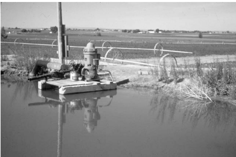
Fig. 8 A typical tailwater recovery and reuse facility. (Utah State University Irrigation Photo Archives.)
