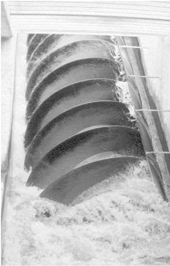
Fig. 2 Archimedes' water screw in its modern form, as implemented in the wastewater treatment plant of Athens (one of nine screws that pump 1 million m 3 per day).
