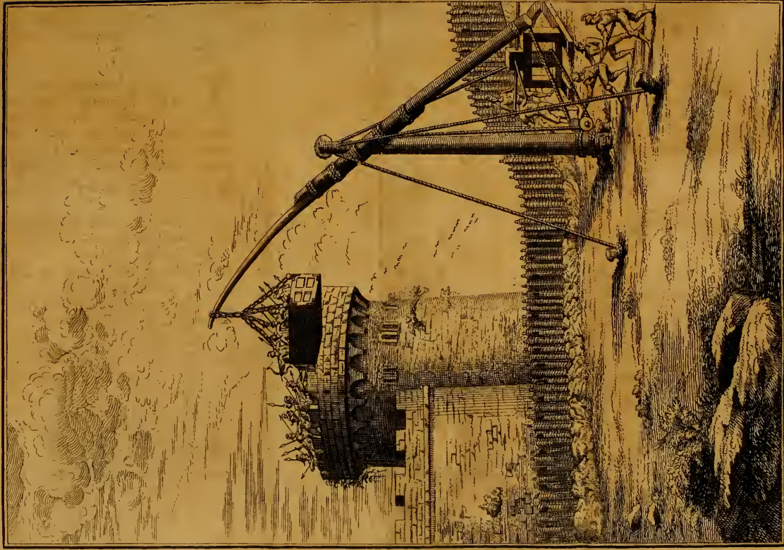
Corvus (or Crane) with a Cage or the Tellenum used by the Ancients for lifting men to the top of works.
