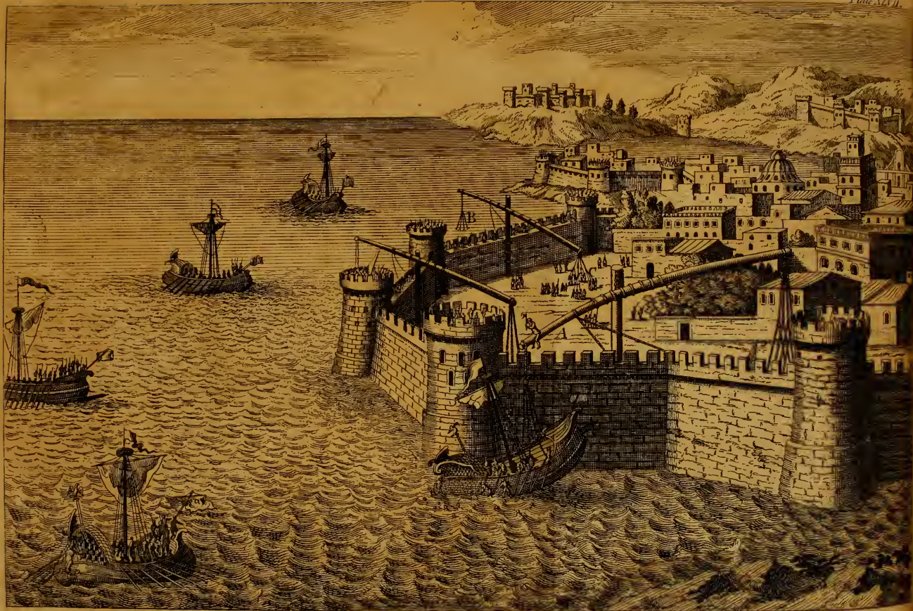
Corvus (or Crane) of Archimedes according to Polybius and Plutarch for seizing and lifting Ships out of the Water
