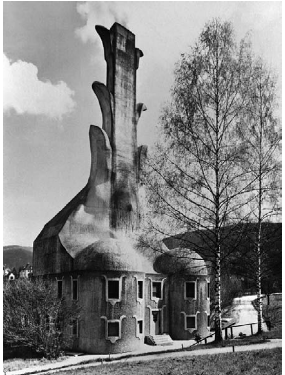
Expression of the forces at work in boiler and flue: boilerhouse at the Goetheanum, Switzerland.
