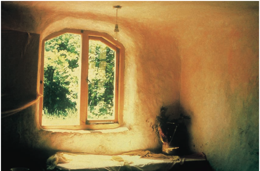
This room was exactly square, gloss-smooth rendered with 3:1 cement:sand(!) – uninhabitable! Softening its textures, plane-meetings and lazure painting it in transparent glowing colours, transformed its mood.
