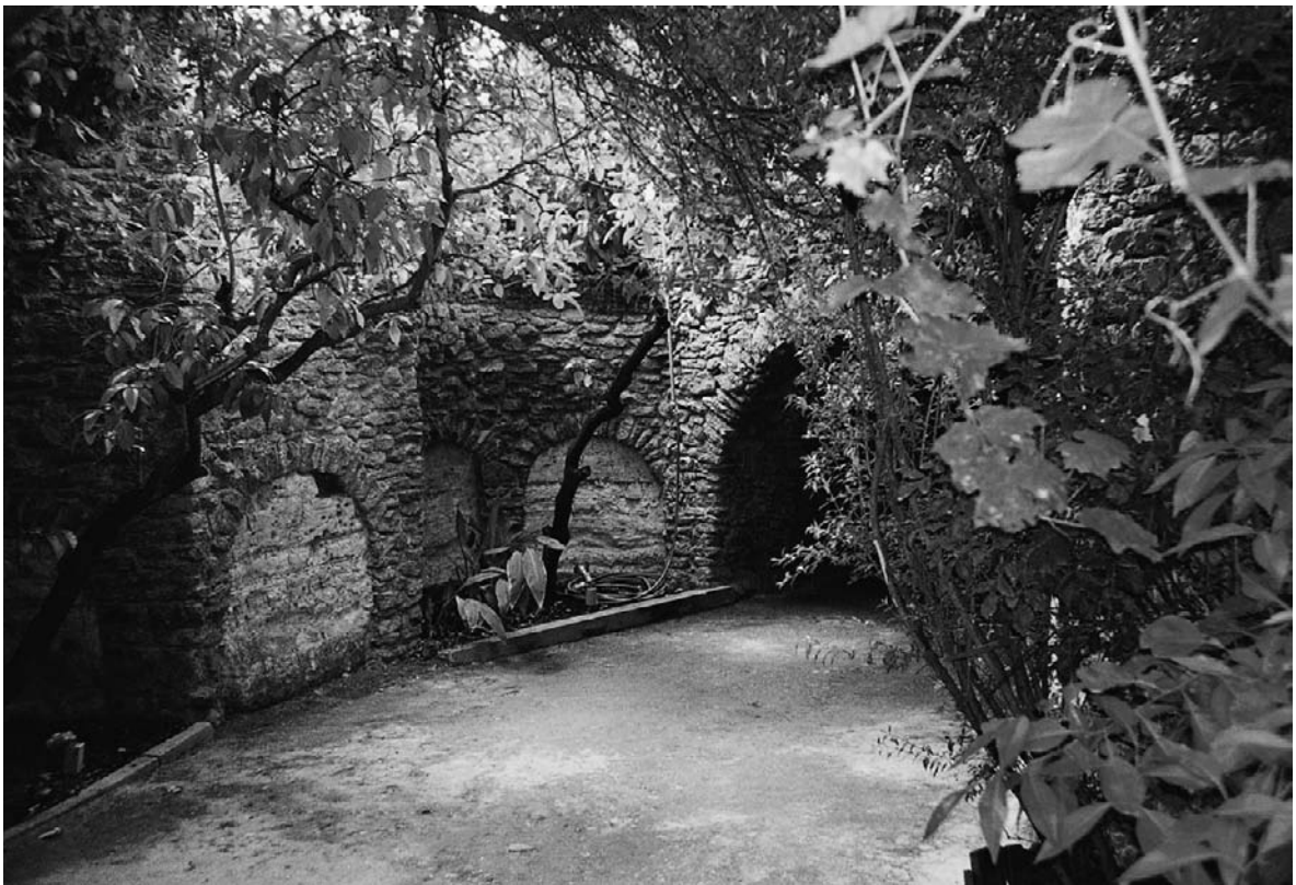
Underground gardens, Fresno, California by Baldesare Forestiere. The massive cooling reserve is replenished nightly by cool air 'drainage'.
