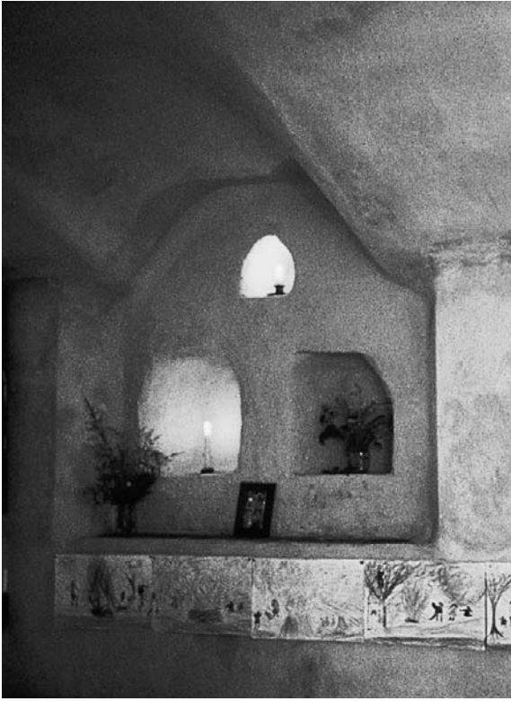
Volunteer work unavoidably involves people – so opportunities for artistic details arise that all too easily get passed over in conventional, non-gift, construction (Wales).
