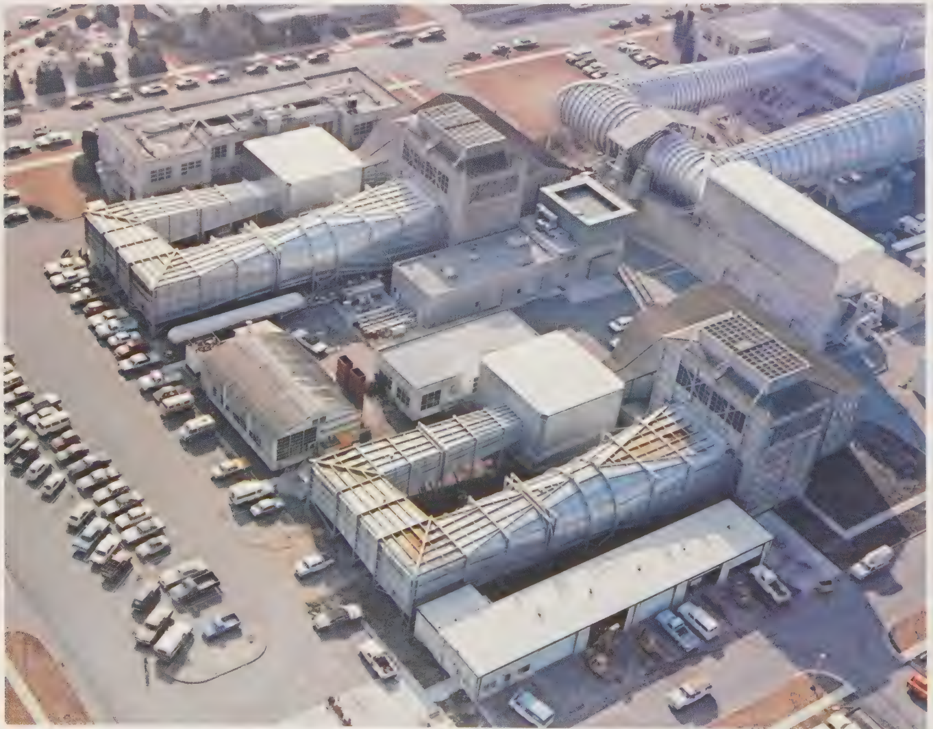
The two wartime 7 \times 10 -foot wind tunnels built at Ames. The test sections are in the blocklike buildings on the left-hand sides of the air circuits.
