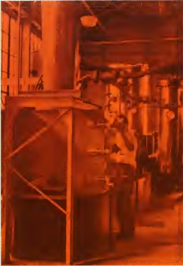
The Langley 11-inch high-speed tunnel. High-pressure air being discharged from the nearby variable density tunnel was injected at an annular port immediately downstream from the test section. Entraining still or low-speed air in the tunnel, the injector pulled tunnel air along with it at high velocities. Speeds near Mach 1 were attained in the test section, but test durations usually lasted only about 1 minute.
