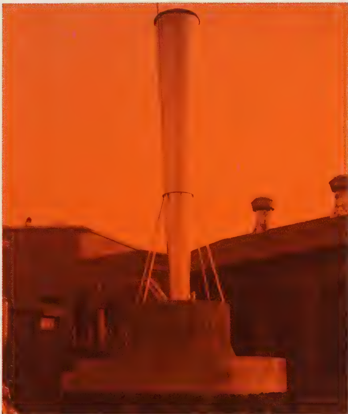
The 24-inch high-speed tunnel also relied on the variable density tunnel for high-pressure air. Shown here outside the variable density tunnel building at Langley, the 24-inch tunnel, like the earlier 11-inch high-speed tunnel, was mounted vertically.
