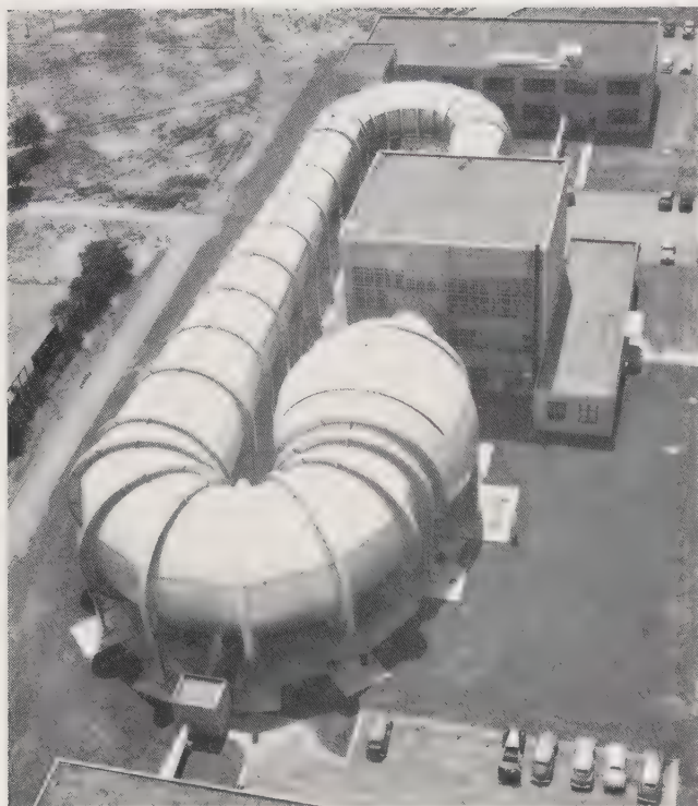
High-speed air circulating in the 12-foot pressure tunnel is turned by several angular stages rather than a single 90 degree corner. The spherical bulge houses the antiturbulence screens.
