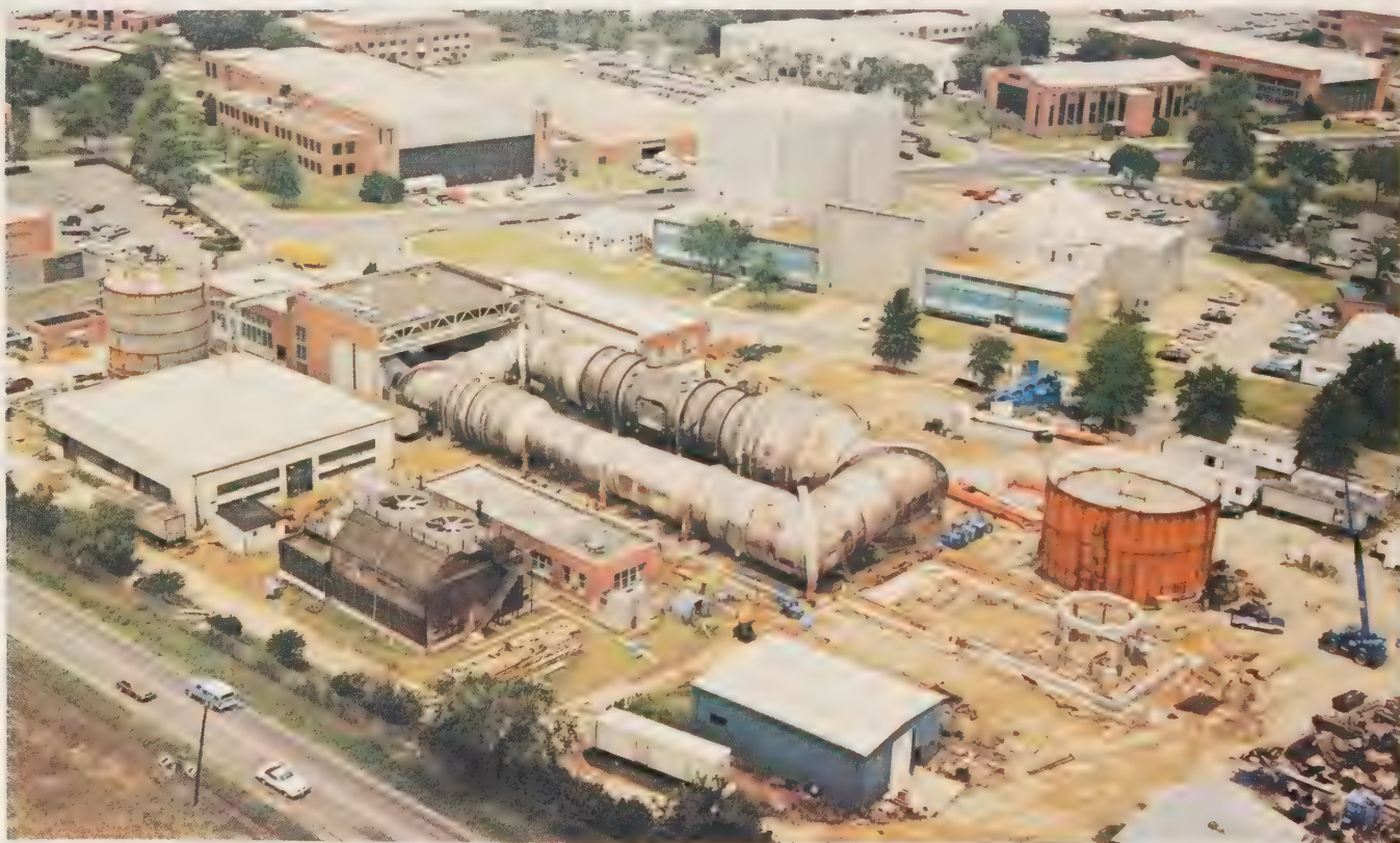
The National Transonic Facility under construction at Langley in 1980.
