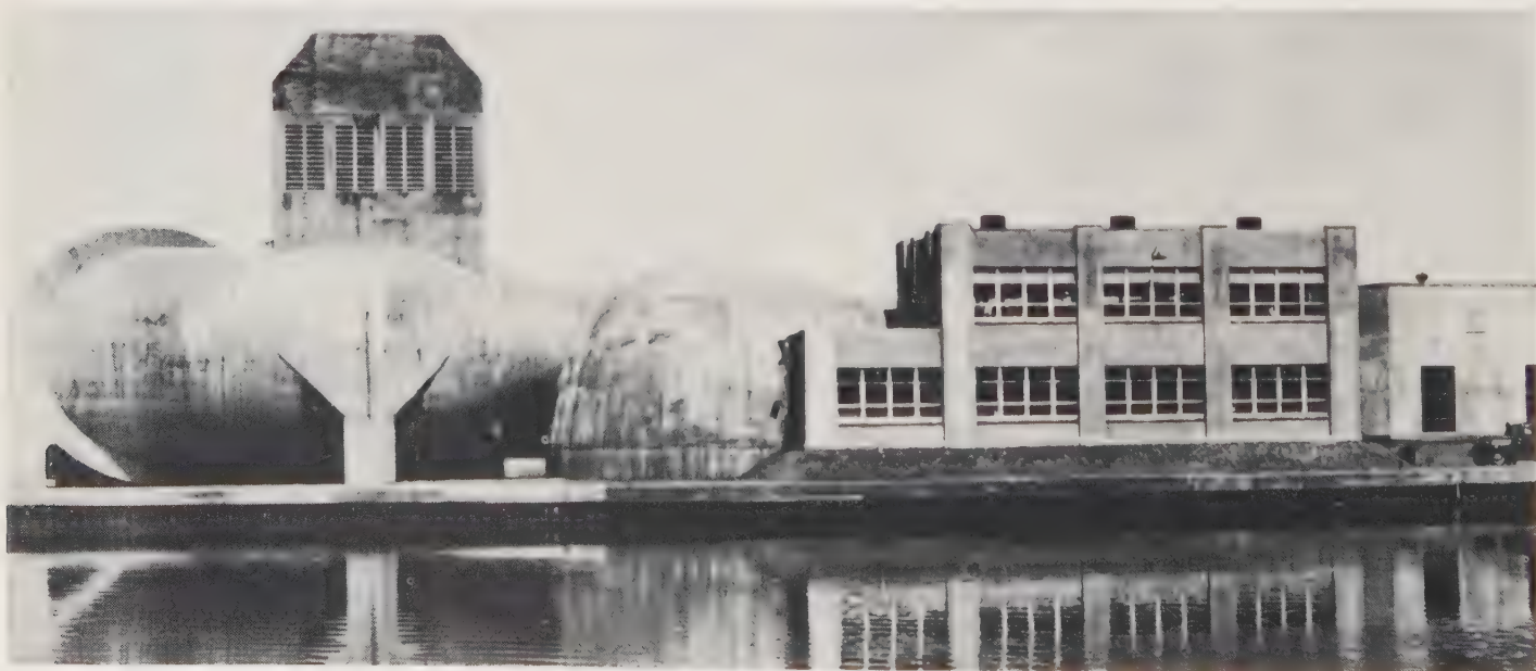
The Langley 8-foot high-speed tunnel. The test section was housed in the concrete igloo. A heat exchanger is shown above the tunnel. This was necessary to remove the large quantities of heat generated by the big fan.
