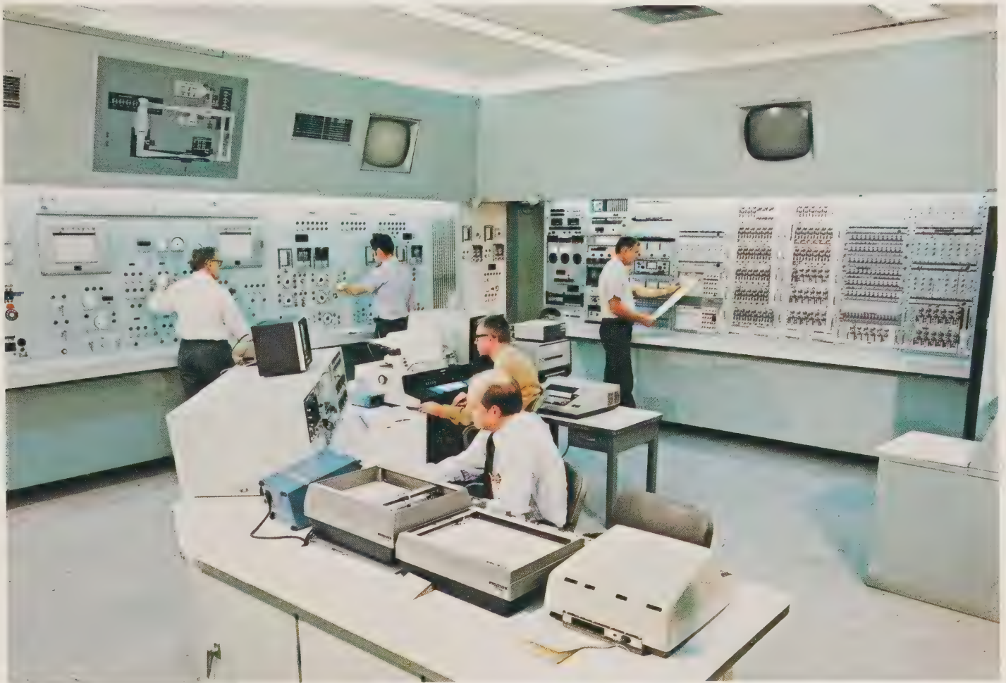
Control consoles for the Lewis 10 × 10-foot supersonic wind tunnel, 1980.
