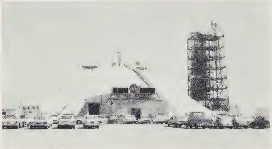
Fig. 8-8. View of a large blockhouse at Cape Kennedy. (NASA photograph)
