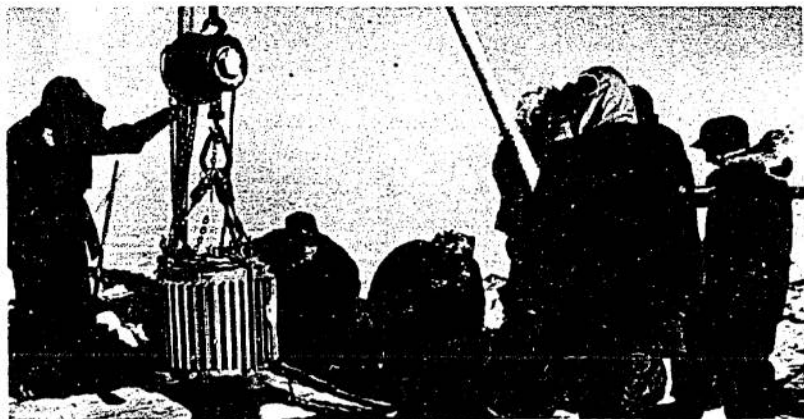
Installing a SNAP-7C radioisotope generator in the ice 700 miles from the South Pole. It provided power for an unattended weather station.
