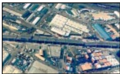
The collapsed section of the Nimitz Freeway.
