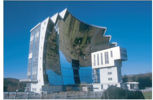
Figure 245 The last mirror of the solar furnace at Odeillo, in the French Pyrenees (© Gerhard Weinrebe)
