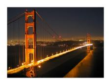
w / The Golden Gate Bridge's roadway is held up by the tension in the vertical cables.
