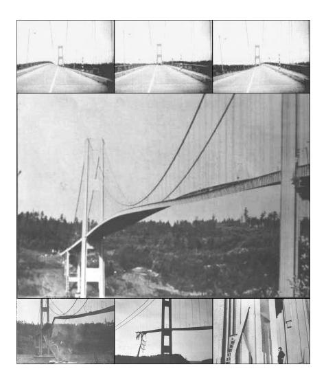
*Top:* A series of images from a film of the Tacoma Narrows Bridge vibrating on the day it was to collapse. *Middle:* The bridge immediately before the collapse, with the sides vibrating 8.5 meters (28 feet) up and down. Note that the bridge is over a mile long. *Bottom:* During and after the final collapse. The right-hand picture gives a sense of the massive scale of the construction.
