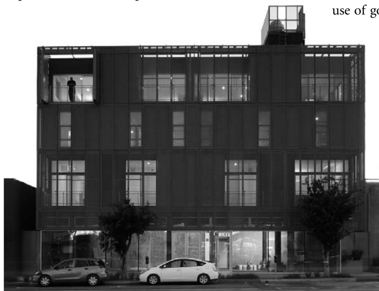
Cherokee Mixed-Use Lofts is an urban market-rate housing project and was the first LEED-certified building in Hollywood, California.
