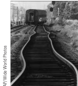
(Example 10.3) Thermal expansion: The extreme heat of a July day in Asbury Park, New Jersey, caused these railroad tracks to buckle.
