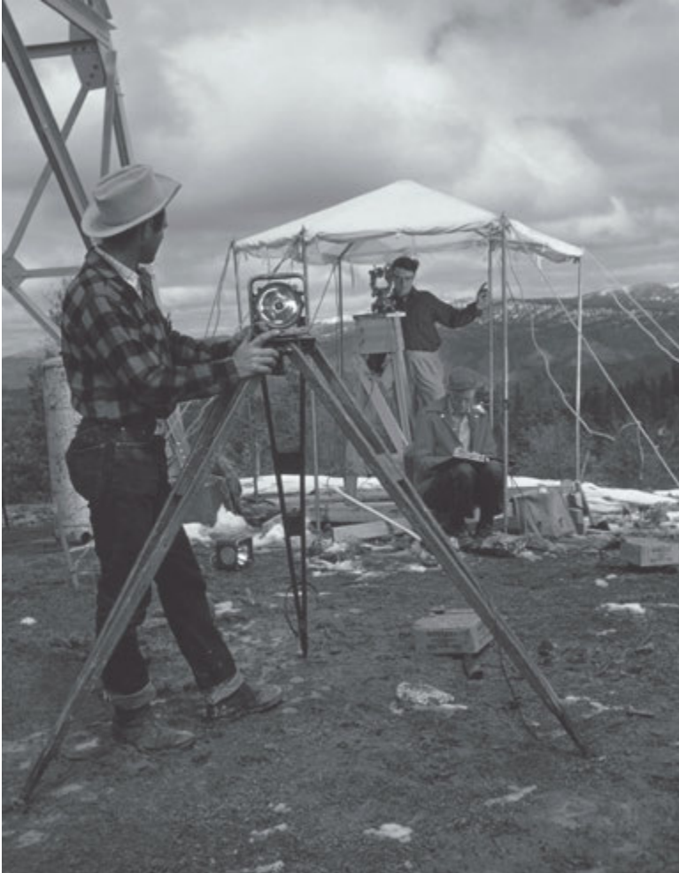
Two surveyors with a theodolite take triangulation readings. J. Baylor Roberts/National Geographic/Getty Images
