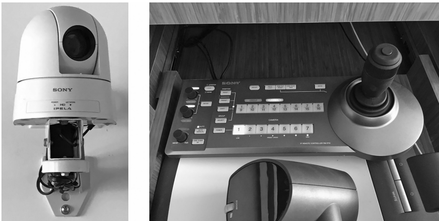
FIGURE 5.2 The camera is attached to the rear wall of the classroom and controlled by a joystick/keypad device located in a cabinet located inside a podium at the front of the classroom.
