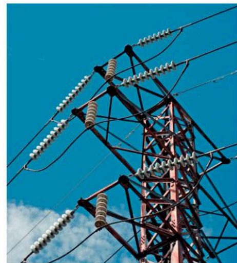
▲ Figure 14.1.4 High-voltage insulators used for high-voltage power transmission are made from glass, porcelain or composite polymer materials. Porcelain insulators are made from clay, quartz or alumina and feldspar, and are covered with a smooth glaze to shed dirt.
