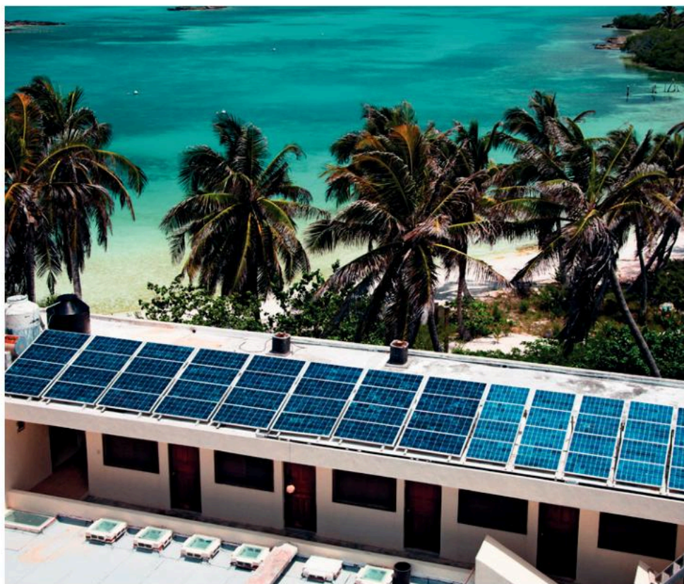
▲ Figure 7.9.9 Photovoltaic or solar cells convert light energy directly into electrical energy. Some panels are turned during the day so that they follow the Sun and receive the maximum amount of light. Large panels can generate high voltages if many groups of cells are connected together in series. Larger currents at lower voltages are possible when many cells are connected together in parallel.
