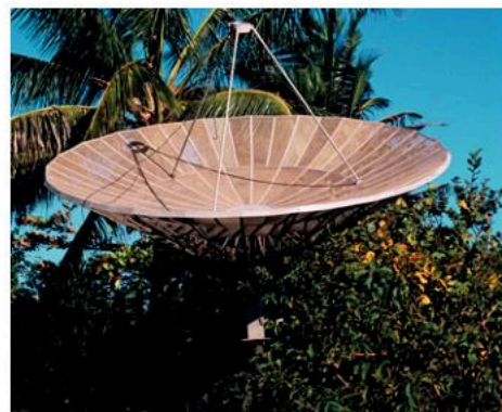
▲ Figure 12.4.2 The metal mirrors focus microwaves onto a small aerial at the focus of the parabolic dish and transmit or receive digital information such as telephone calls.
