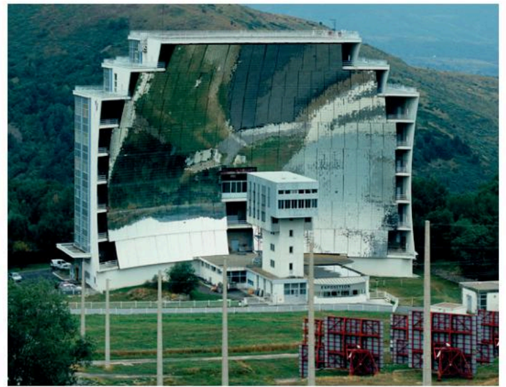
▲ Figure 7.11.4 The French solar furnace in Odielle in the Pyrenees uses over 20 000 electronically controlled mirrors to reflect the Sun's radiation energy into a furnace housed in the building at the focus of the mirrors. The temperature in the furnace can quickly reach over 3000^\circ\text{C} .
