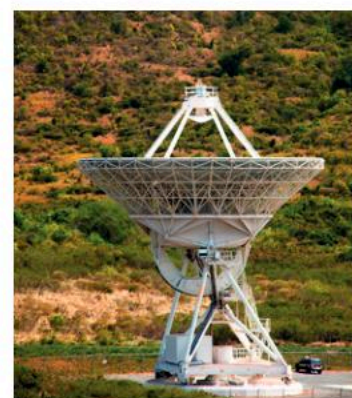
▲ Figure 7.9.7 Signals arriving at the satellite are very weak and a large collecting surface is needed to detect them. Electrical energy supplied to the satellite is used to amplify the signals before they are re-transmitted.
