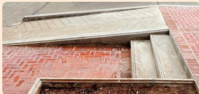
▲ This ramp enables wheelchair access
