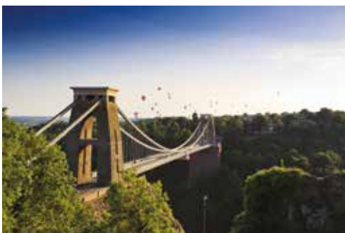
The cables from a suspension bridge
